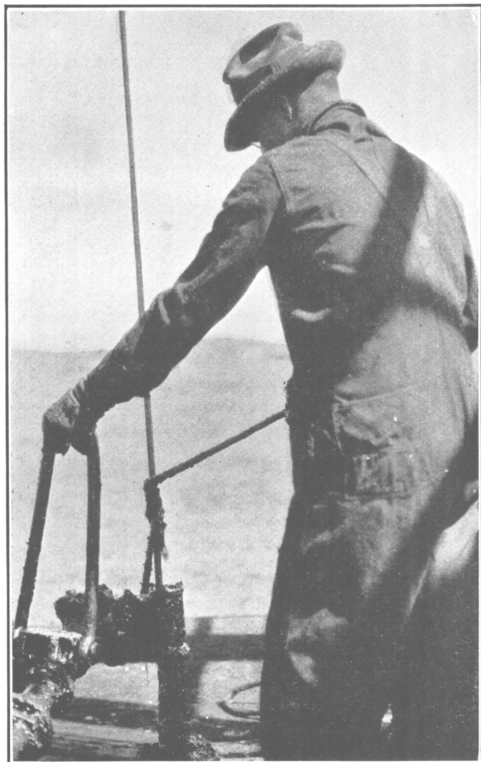
FIGURE 24.—Safe method of stripping paraffin from sucker rods
