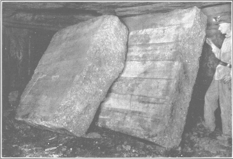
FIGURE 35.—Débris of stopping 7, viewed from original position
