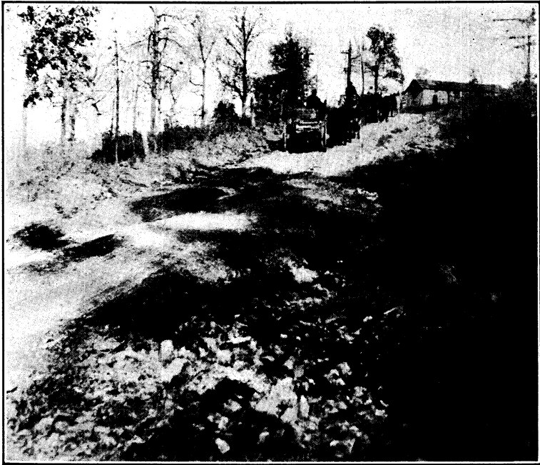
FIGURE 22.—Hauling fluorspar over poor roads in Kentucky
