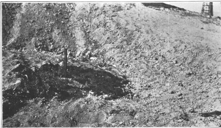
B. SEEPAGE FROM EARTHEN RESERVOIR SHOWN ABOVE.
