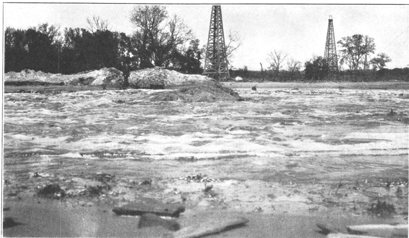
B. CRATER OF MAGNOLIA CO.'S MAYS-NEWBERRY WELL NO. 1, AFTER BLOWING WILD FOR ABOUT THREE MONTHS, AND A RELIEF WELL, ROBBERTSON FIELD, OKLA. (Courtesy of M. J. Kirwan.)
