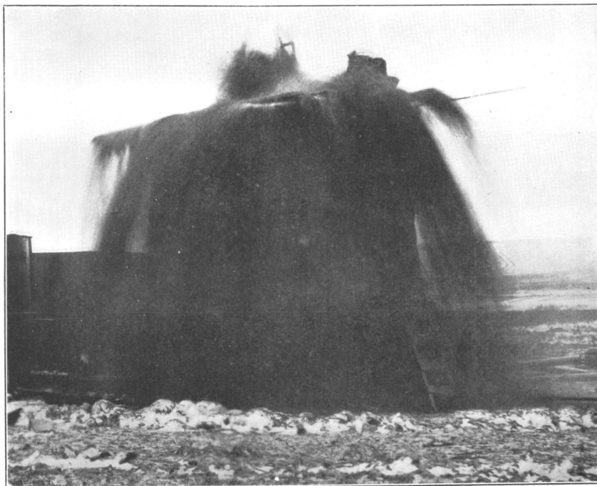
B. WASTE OF OIL AND GAS CAUSED BY FLOWING LARGE WELL INTO SMALL OPEN TANK.
