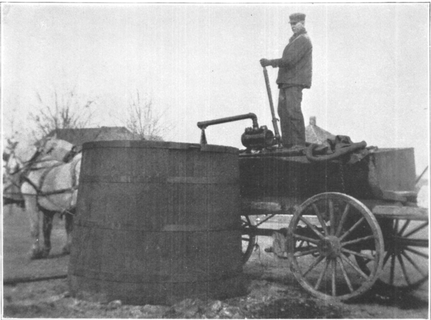
B. PORTABLE PUMPS AND TANK FOR PICKING UP SMALL AMOUNTS OF OIL.
