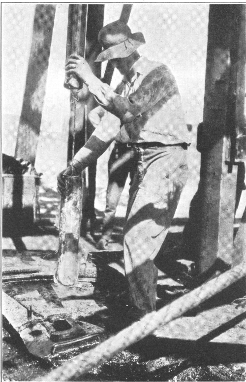
B. LEAD PLUG FOR CAPPING A PLUG OF LATHE CUTTINGS, READY FOR RUNNING INTO THE WELL.
