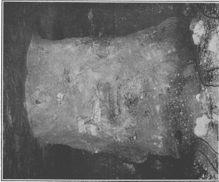
B. PILLAR LEFT TO SUPPORT ROOF OF RELATIVELY HIGH WORKING FACE.
