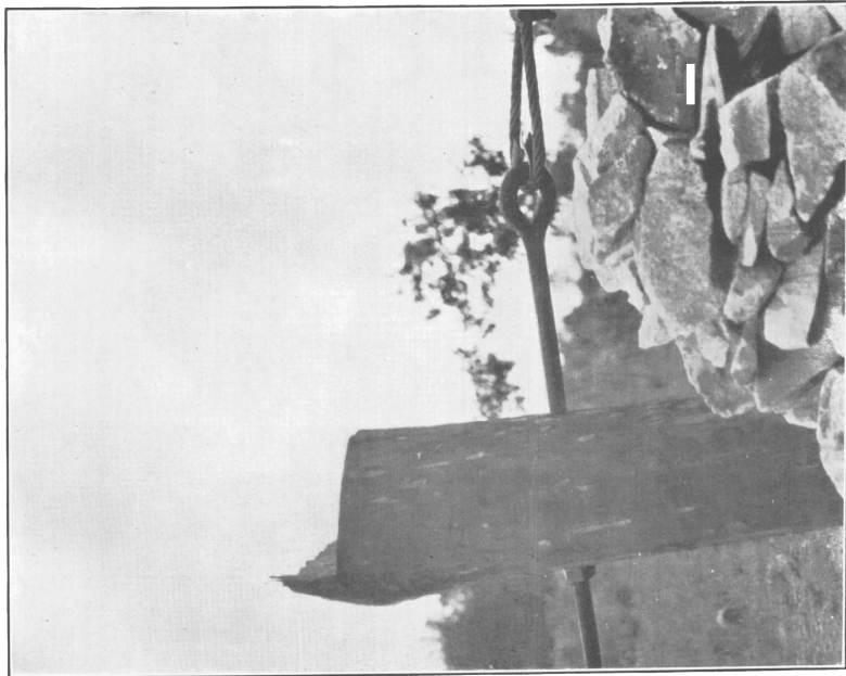
41. A GUY ANCHOR POST USED IN TENNESSEE.
