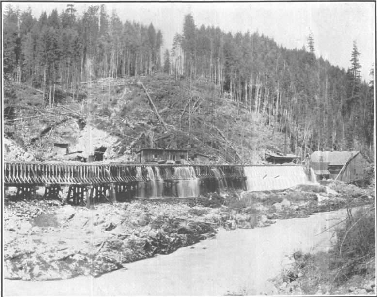
B. POWER HOUSE, PORTAL, AND PART OF FLUME, NISQUALLY TUNNEL, ALDER, WASH.
