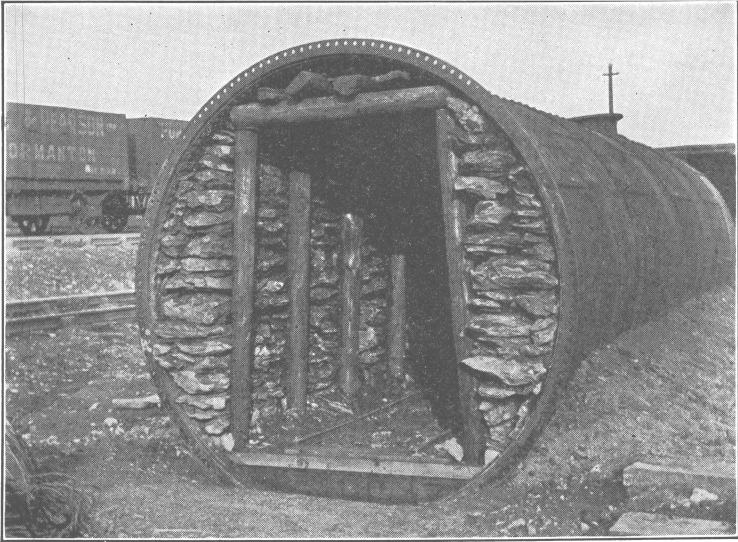
A. TIMBERING AND STONE PACKING IN PRELIMINARY GALLERY AT ALTOFTS.
