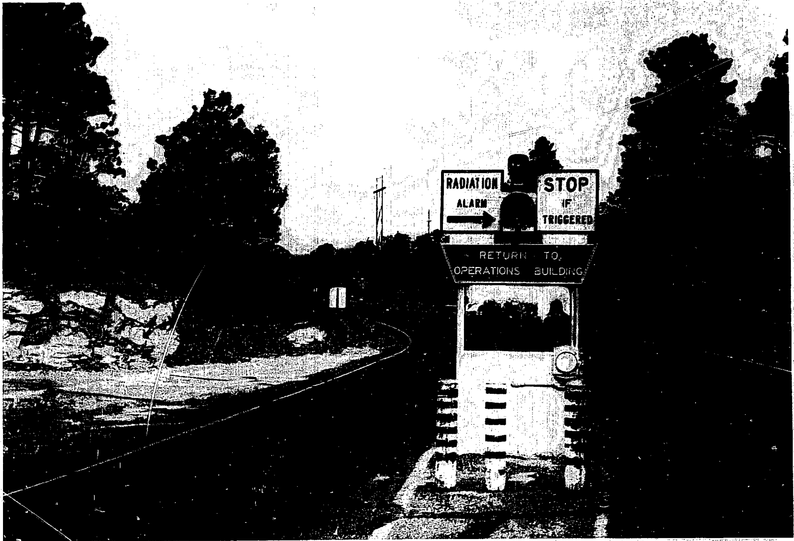
Figure 1. The guard station with alarm light and Klaxon. The system electronics are mounted inside the station.
