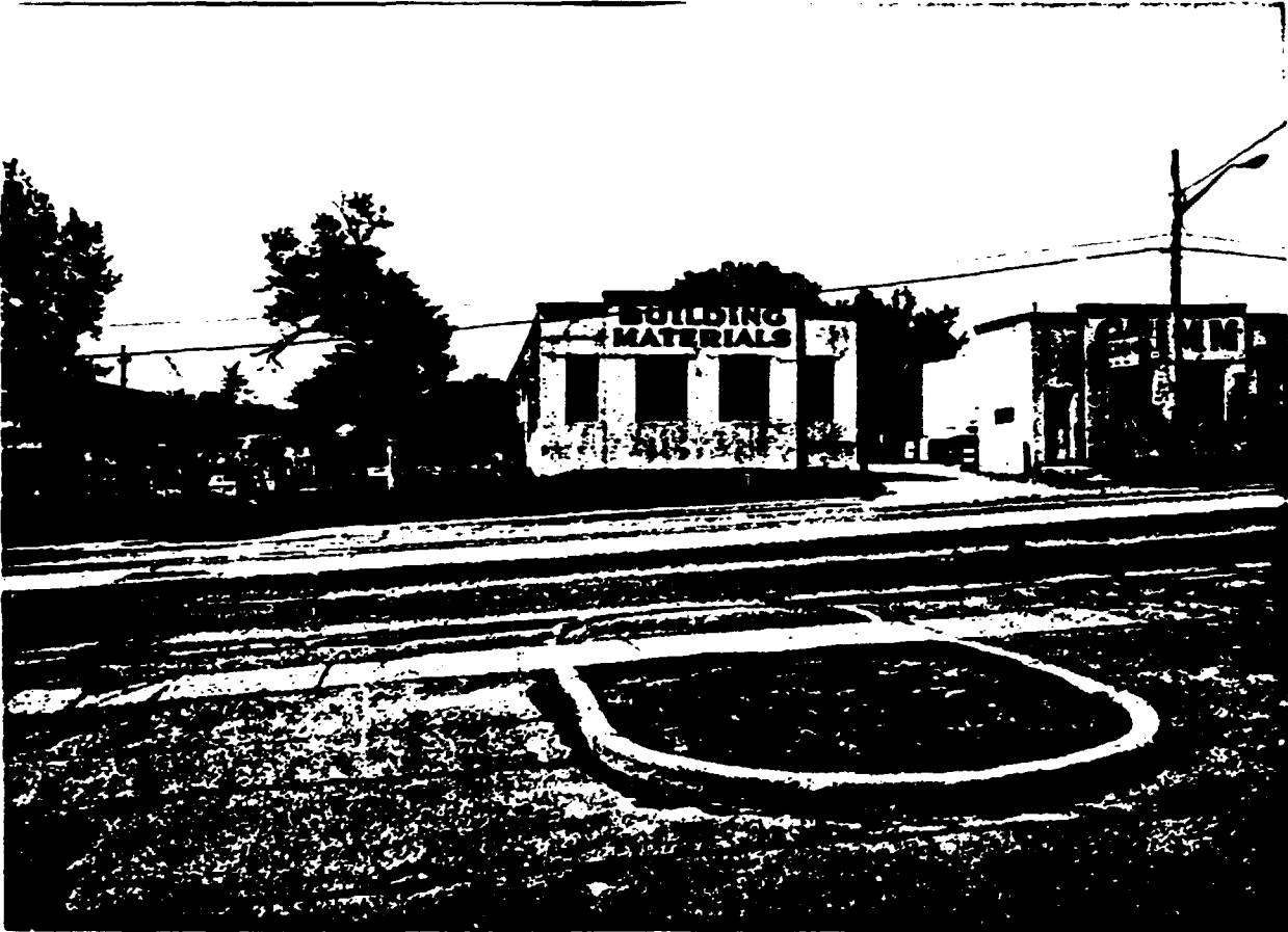
Fig. 2. Front view of the property at 1110 Central Avenue, Albany, New York (AL215) looking southwest.
