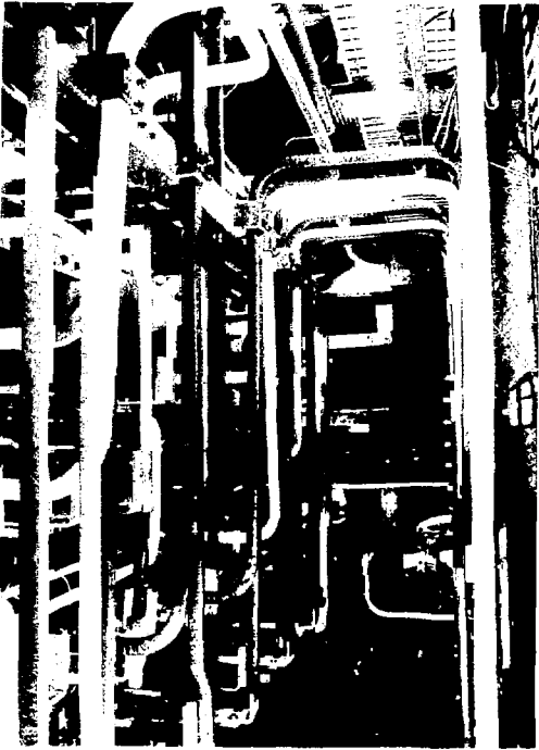
Figure 19. The PBX-M buswork configuration behind the PBX-M switching panels. (B6E0887)
