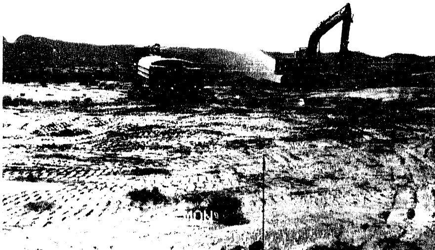
Dust control activities at the southwest side of the processing site at Monument Valley, AZ.
