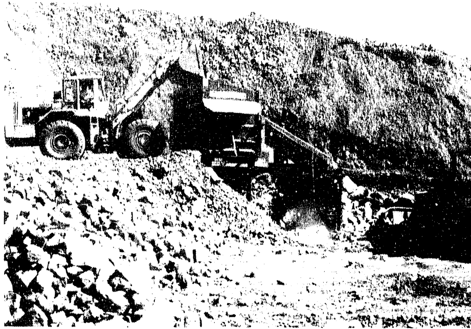
A motorized grizzly, located at the Shear's quarry, is used to produce erosion protection rock (RIPRAP) for the covering of the Lakeview, OR, tailings.
