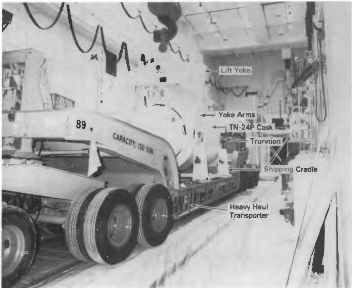
Figure 3-27. Cask with Lift Yoke Attached
