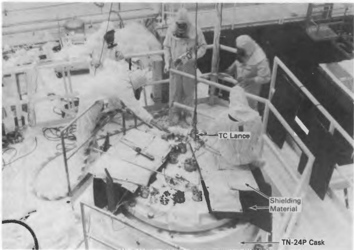
Figure 3-34. Installing thermocouple lances into the fuel assembly guide tubes through the TN-24P test lid.
