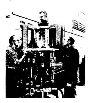
Fig. 8. Skua, a burst-mode critical assembly under construction.
