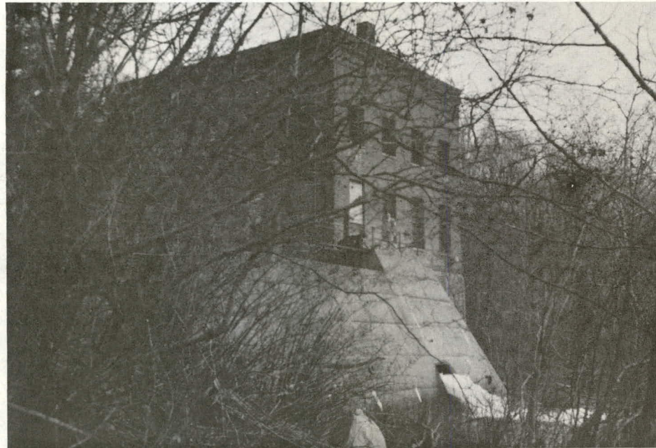
Lower powerhouse looking downstream
