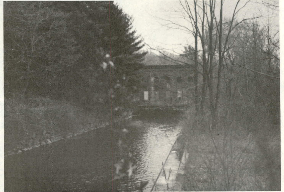
Lower powerhouse and intake channel, looking downstream
