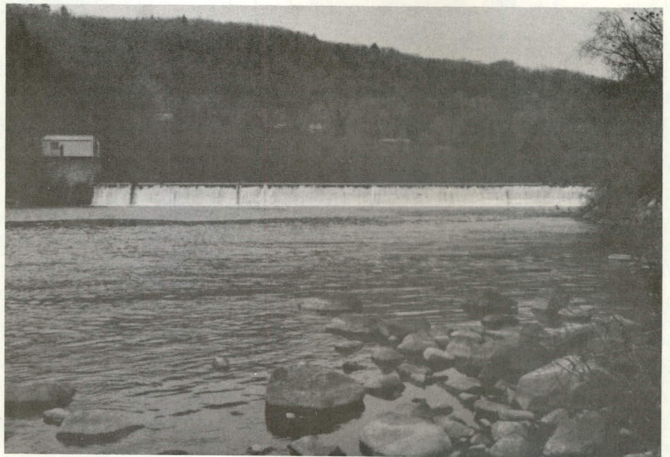
Lower dam looking upstream.
