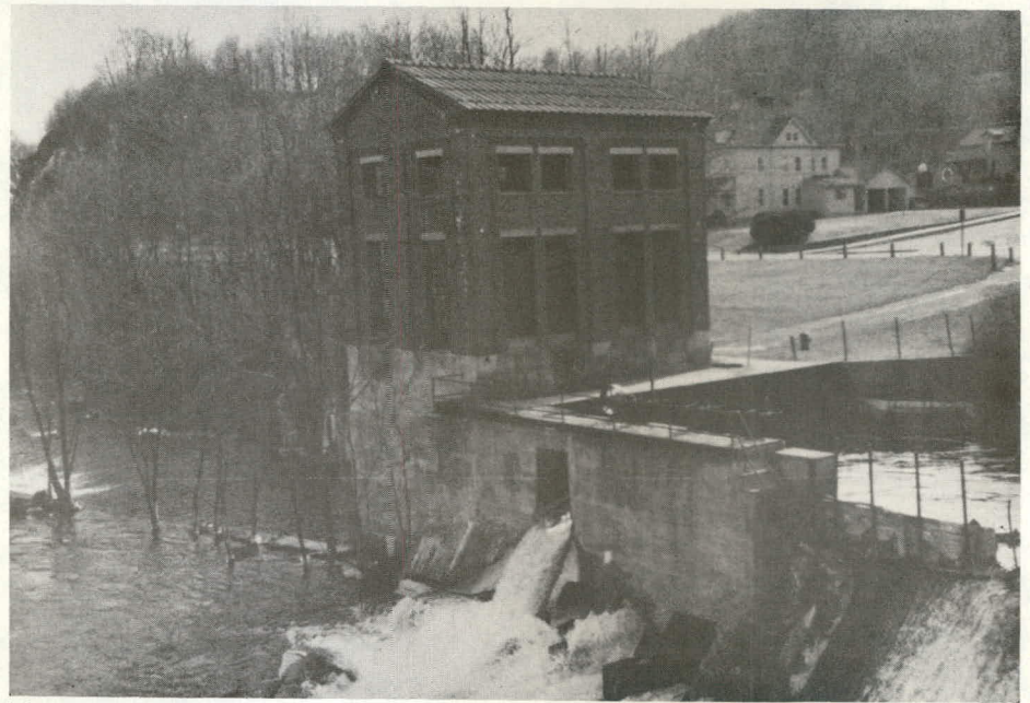
Upper powerhouse and intake from Route 179 Bridge looking southwest.
