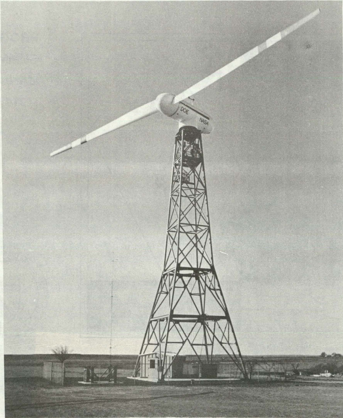
MOD-0A 200 kilowatt wind turbine and meteorological tower at Clayton, New Mexico field-test site.
