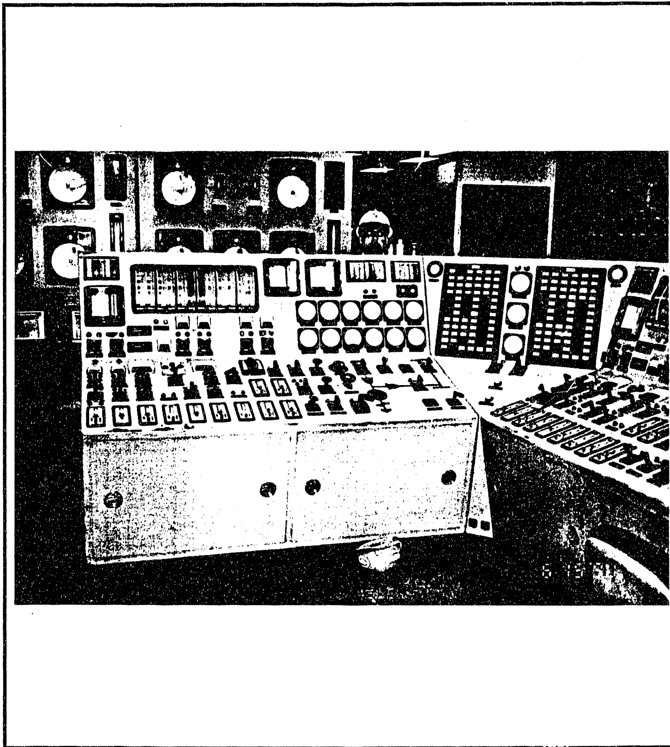
Figure 35. Existing Control Panel Prior to Modification
