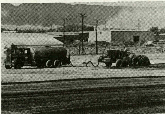
Figure 58. Hydrostatic Stabilizer Mixes Asphalt Emulsion With Tailings
