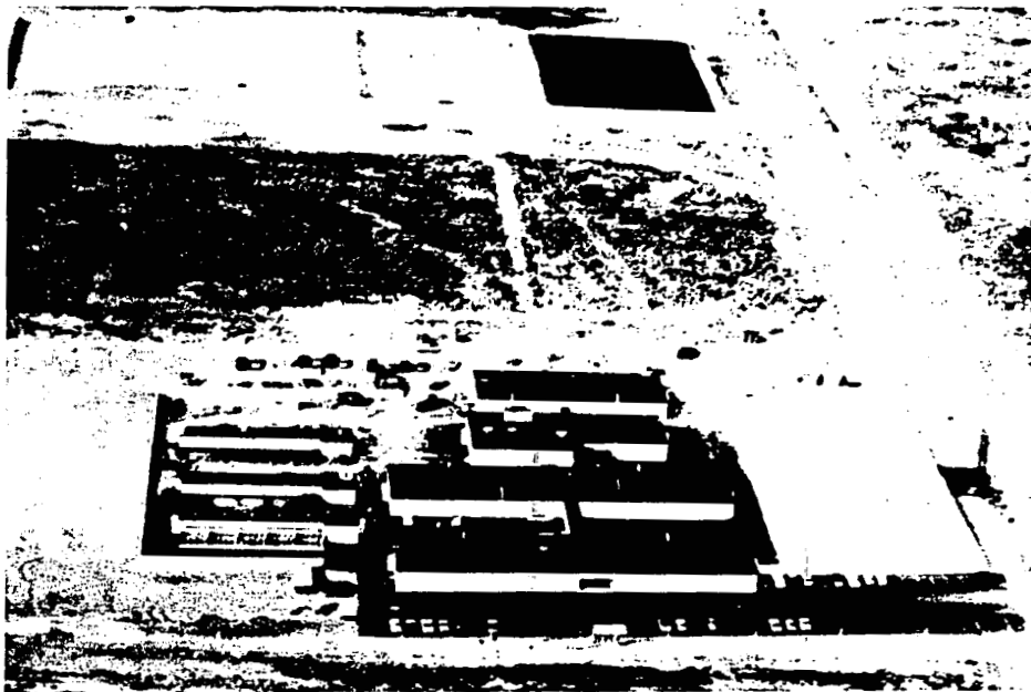
FIGURE 9.28C. The Lovelace project in August 1963, not too long after the inhalation exposure work had been moved out to the Sandia Base. Note the single holding pond at the upper right. This held weakly contaminated water and utilized the strong evaporative power of the desert sun to reduce greatly the volume of material needing disposal. The project was referred to then as the "MEC-1013 Project" or just the "1013" Project.
