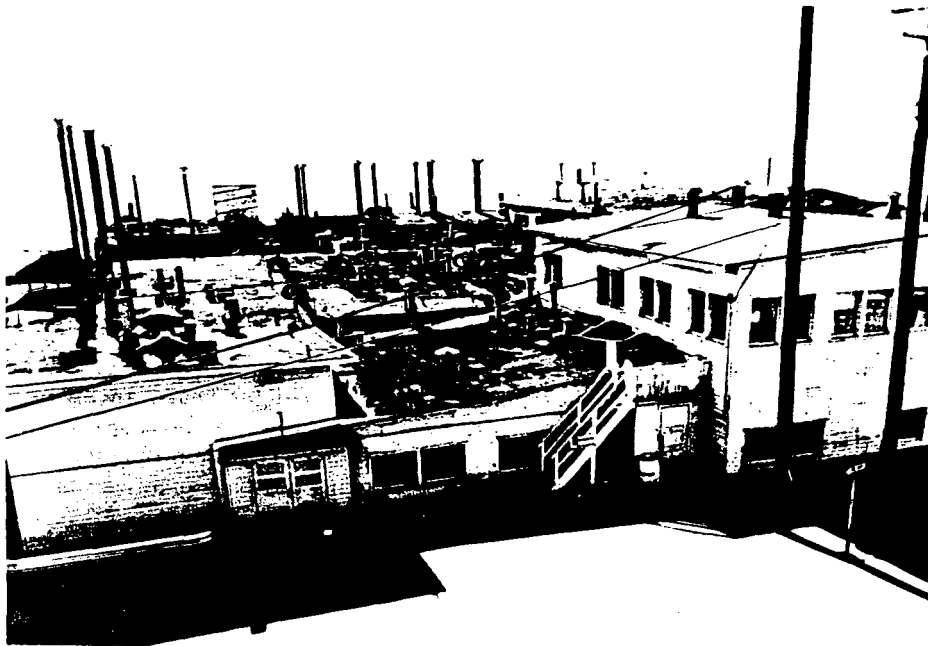
FIGURE 8.14B. View of the "D" Building at Los Alamos in which much of the plutonium metallurgy and chemistry were done. Note that only some of the exhaust stacks are suitably far above the roof line. (Photo courtesy of Dr. George Voelz, Los Alamos.)
