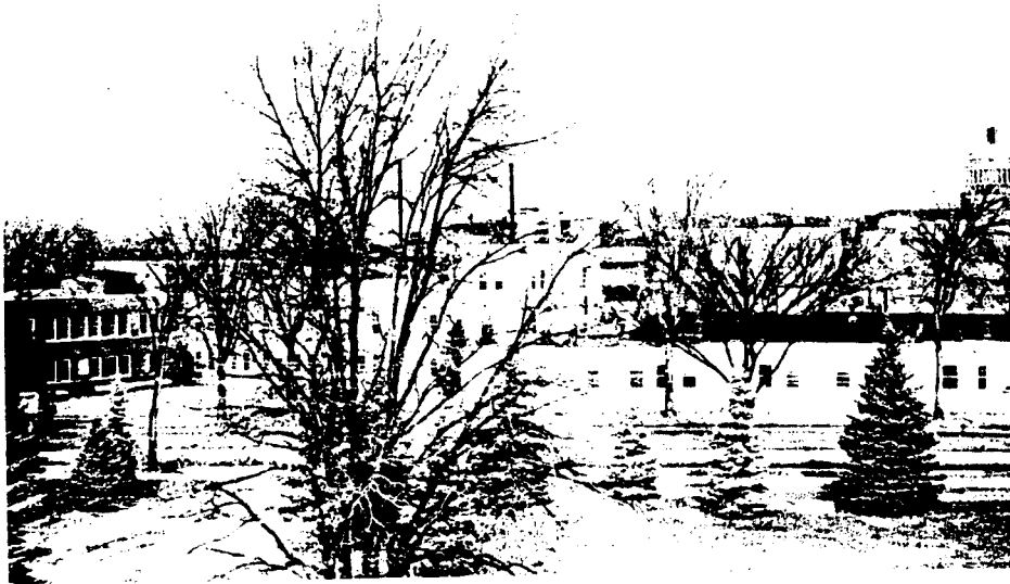
FIGURE 2.1. Early view of the "temporary" buildings housing the MED work at the University of Rochester Medical Center. The one-story building at the right included the animal colony and most of the inhalation exposure chamber. Note that as many as 350 people worked in this facility, about half of them on the uranium work, on eight-hour shifts around the clock. (Courtesy of University of Rochester Medical Center Photographic Unit.)
