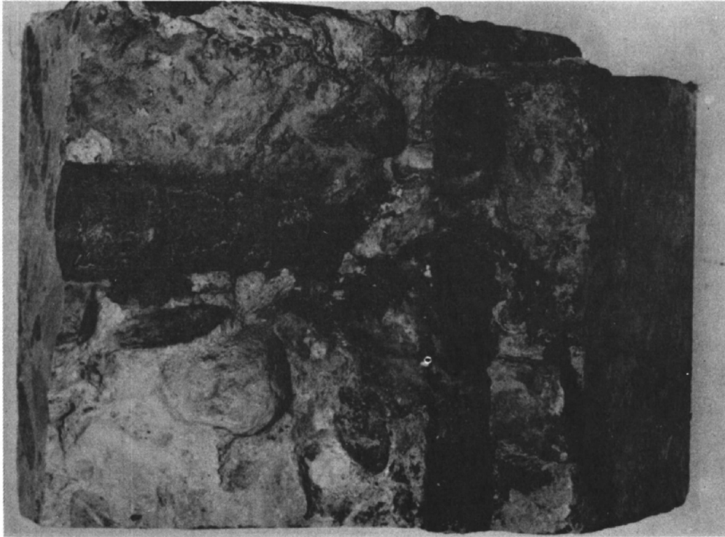
Figure VII-8. Photograph of reinforced pipe section showing staining around rebar. Photo PX-D-60859
