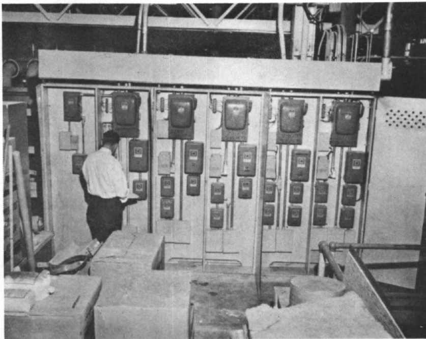
Figure III-11. View showing arrangement of contactors, relays, transformers, etc., used in operation of saline water test equipment. Photo PX-D-60855
