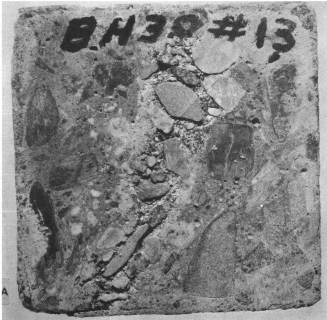
Figure III-18. Concrete containing no available free lime is still susceptible to leaching by hot distilled water. Photo PX-D-55290 NA
