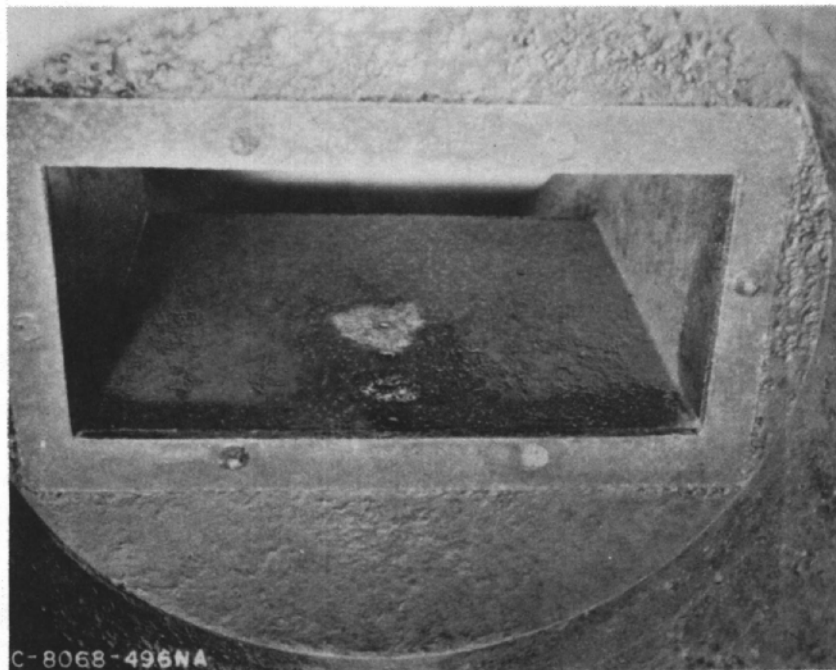
Figure III-64. Concrete orifice after 2 years' subjection to flowing 100° F synthetic sea water. Photo PX-D-60853
