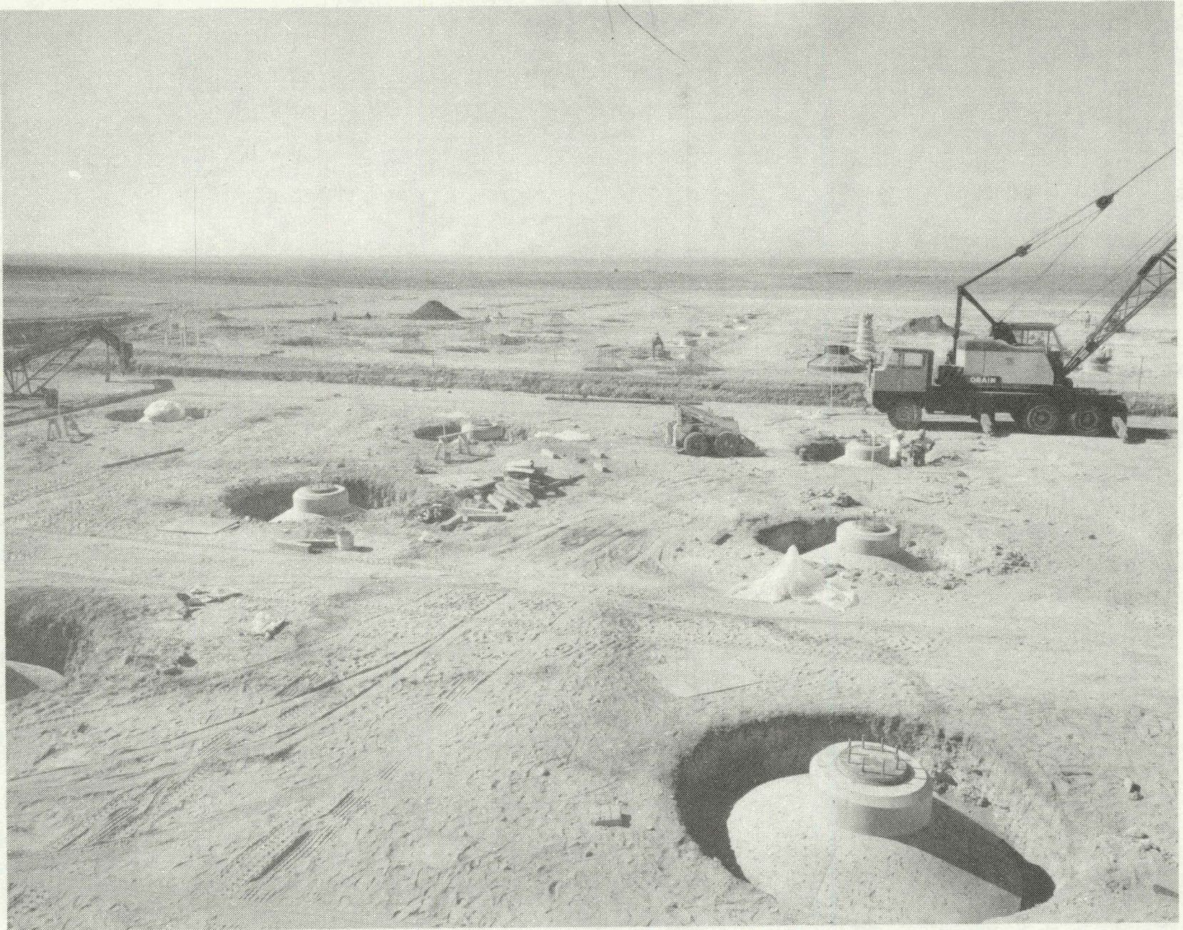
HELIOSTAT FOUNDATION INSTALLATION
