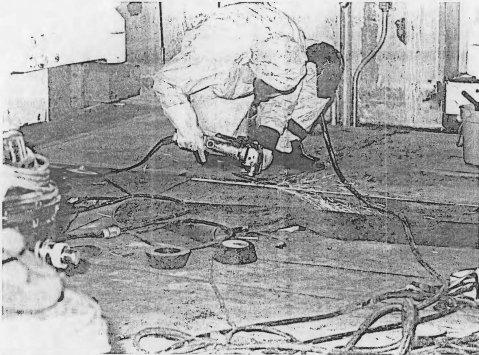
FIGURE 18. Grinding Contamination from Steel Angle-Iron Framework
