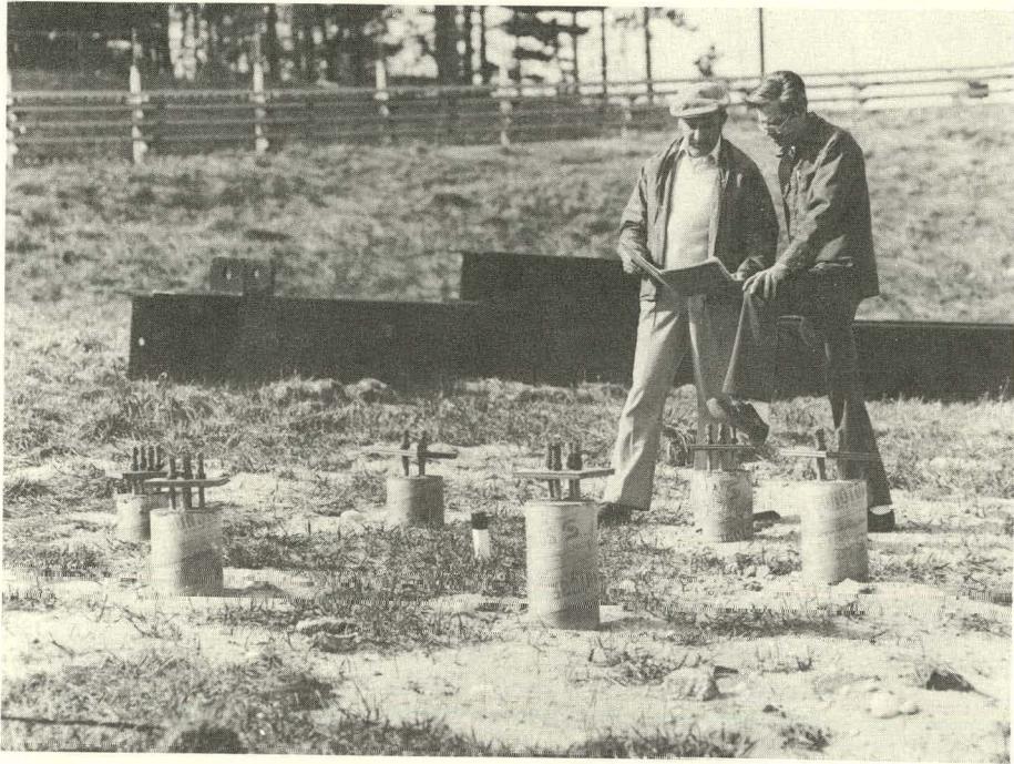
Figure 26. Heliostat footings.
