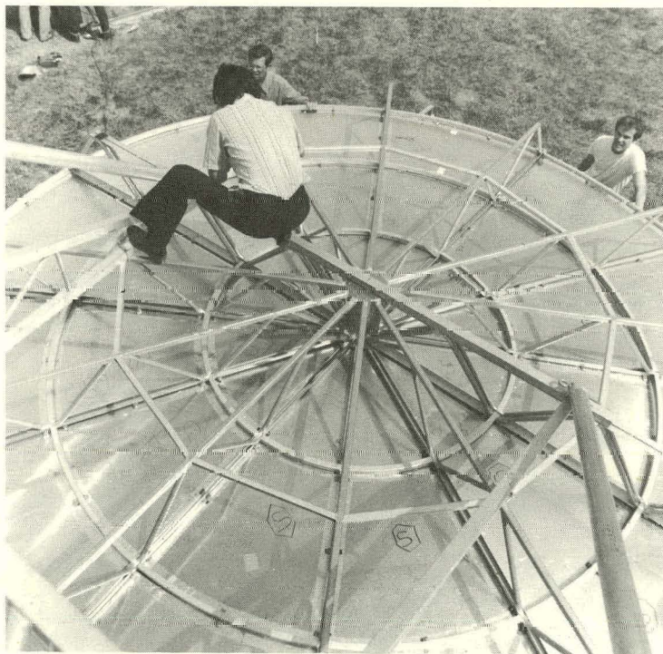
Figure 34. Field assembly of heliostat dish - two halves being bolted back together.
