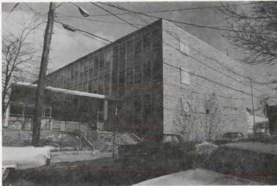
Figure 33. Public School No. 40 View of Building Front
