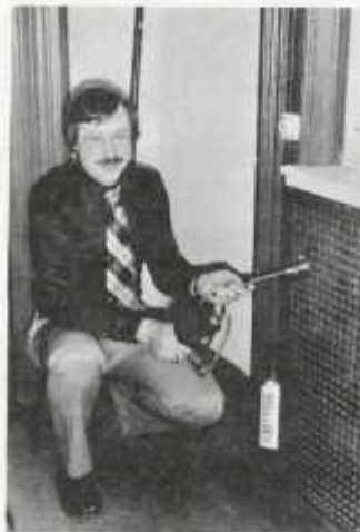
Figure 8. City Hall Cabinet-mounted Radiator with Thermostatic Control Valve Installed
