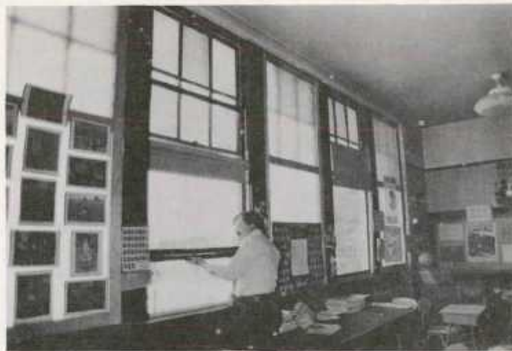
Figure 22. Public School 6 Classroom Windows After Installation of Lexan Plastic Sheet
