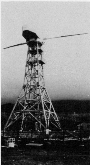
Fig. 11: Japanese 100kW test bed
