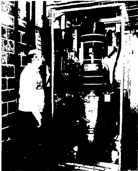
Fig. 7. The 2.45-GHz high-power amplifier with klystron installed. (83E1268)
