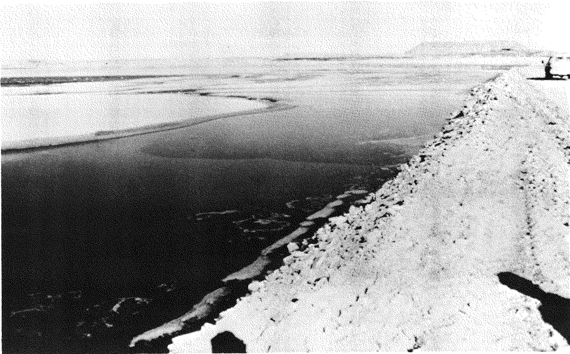
Figure 6. Anaconda Tailings Retention area in Foreground Showing the Southern Embankment and the Solution Pond.
