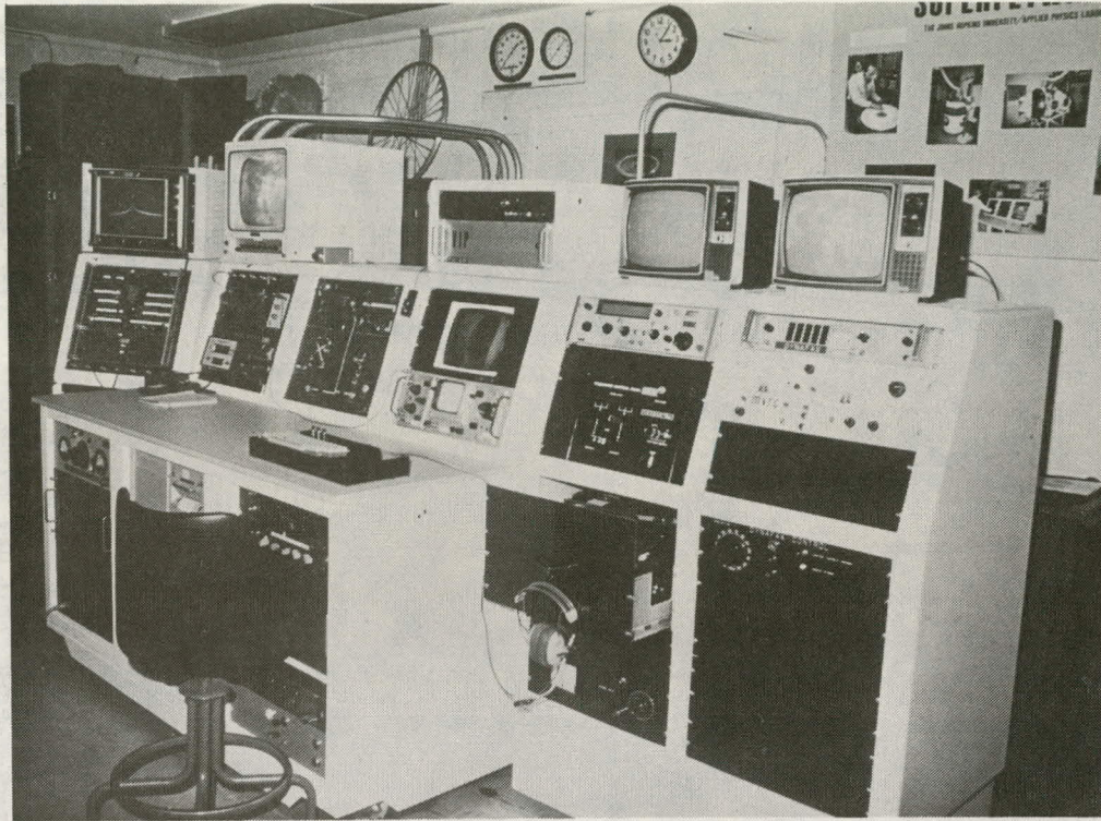
Fig. 5 New control console.
