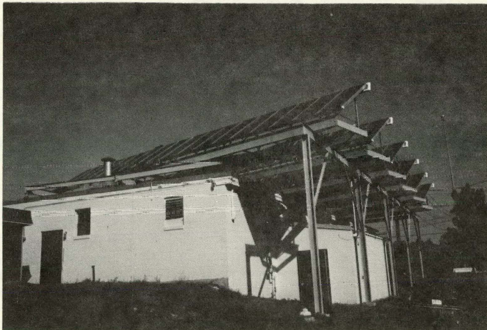
Figure 2. Collector Array, Showing Steel Support Structure Fort Devens Launderette
