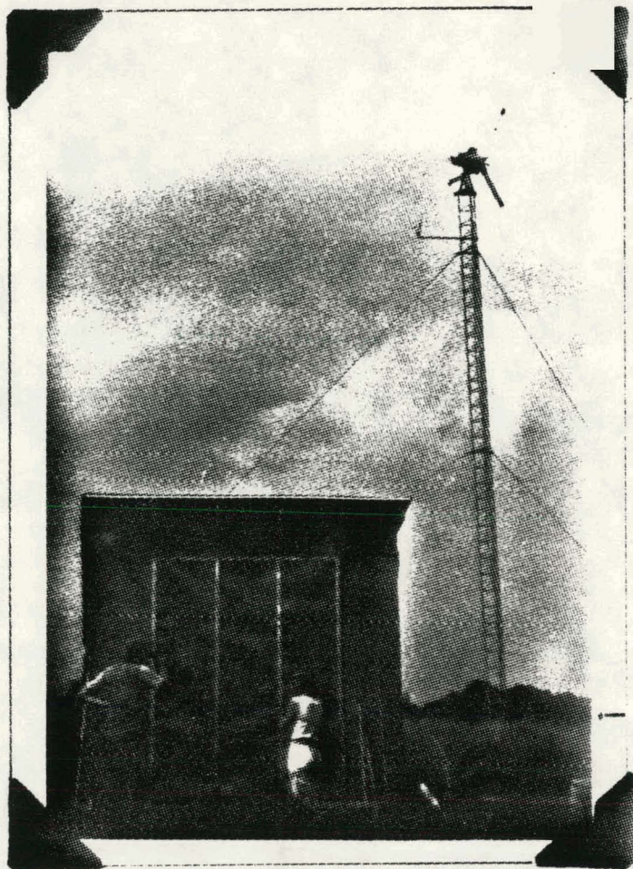
Solar-heated building for battery storage
