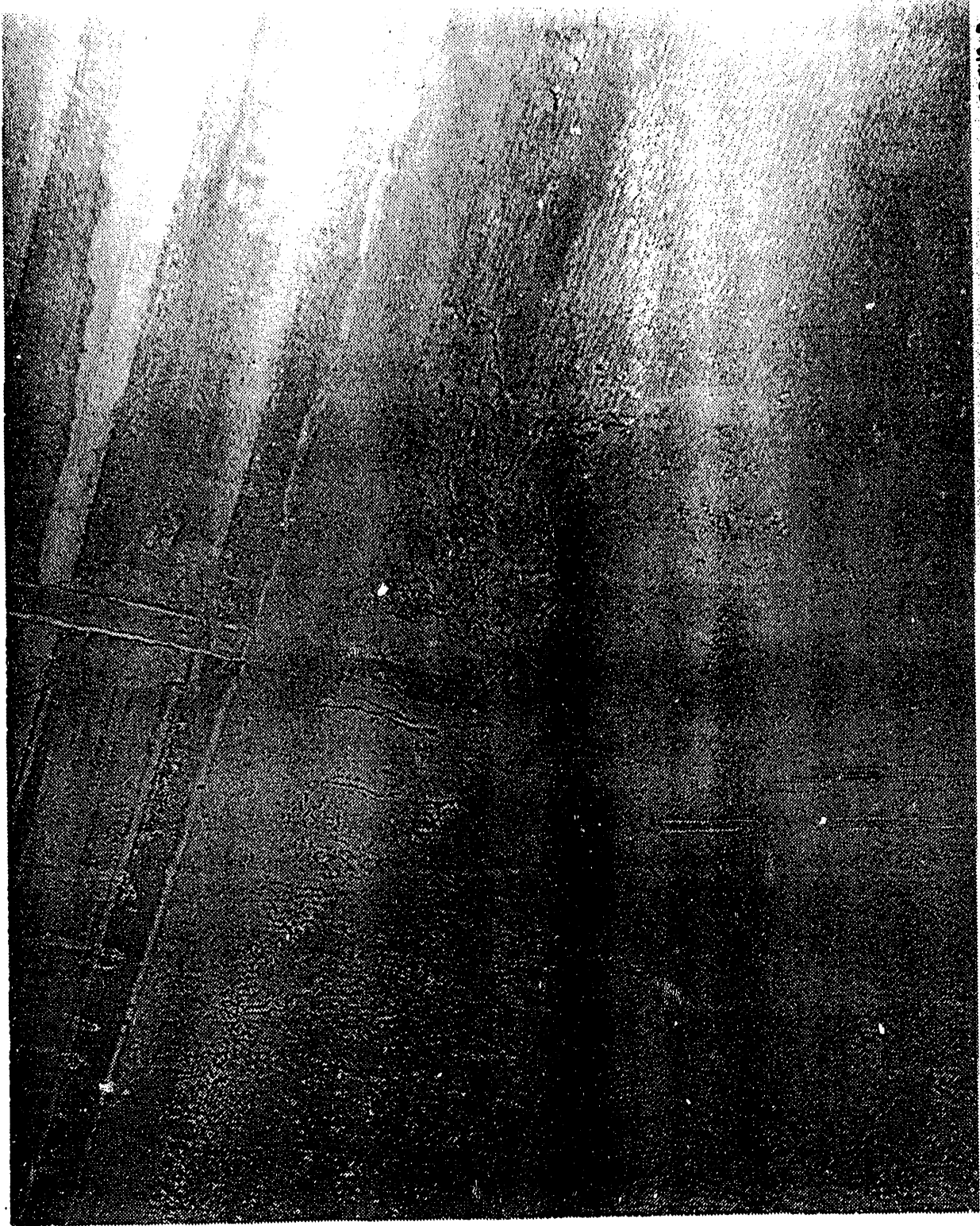
Figure 4. View of Typical Pitting Corrosion Occurring in the Tank Wall at the Liquid Level Interface
