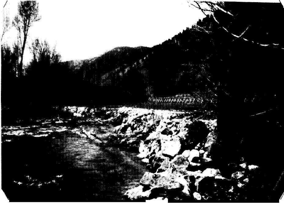
Photo 3: Watershed Stabilization Site 1 (May 1988) just after rock was placed to armor stream bank.
