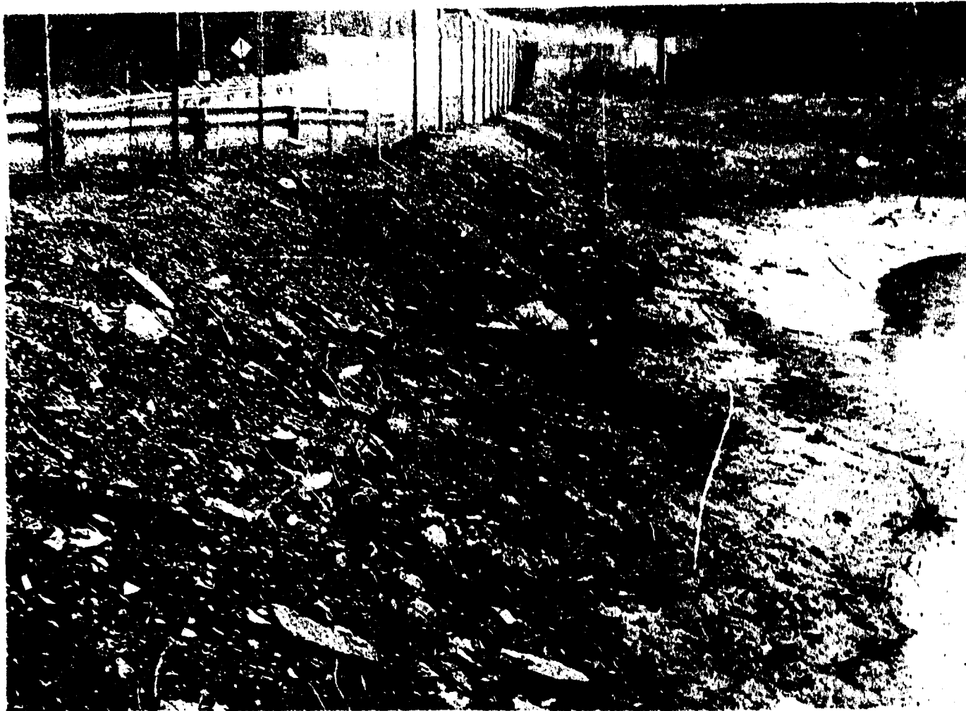
Fig. 2.19. Upstream bed of White Oak Dam (looking north) just after vegetation removal, December 1979.
