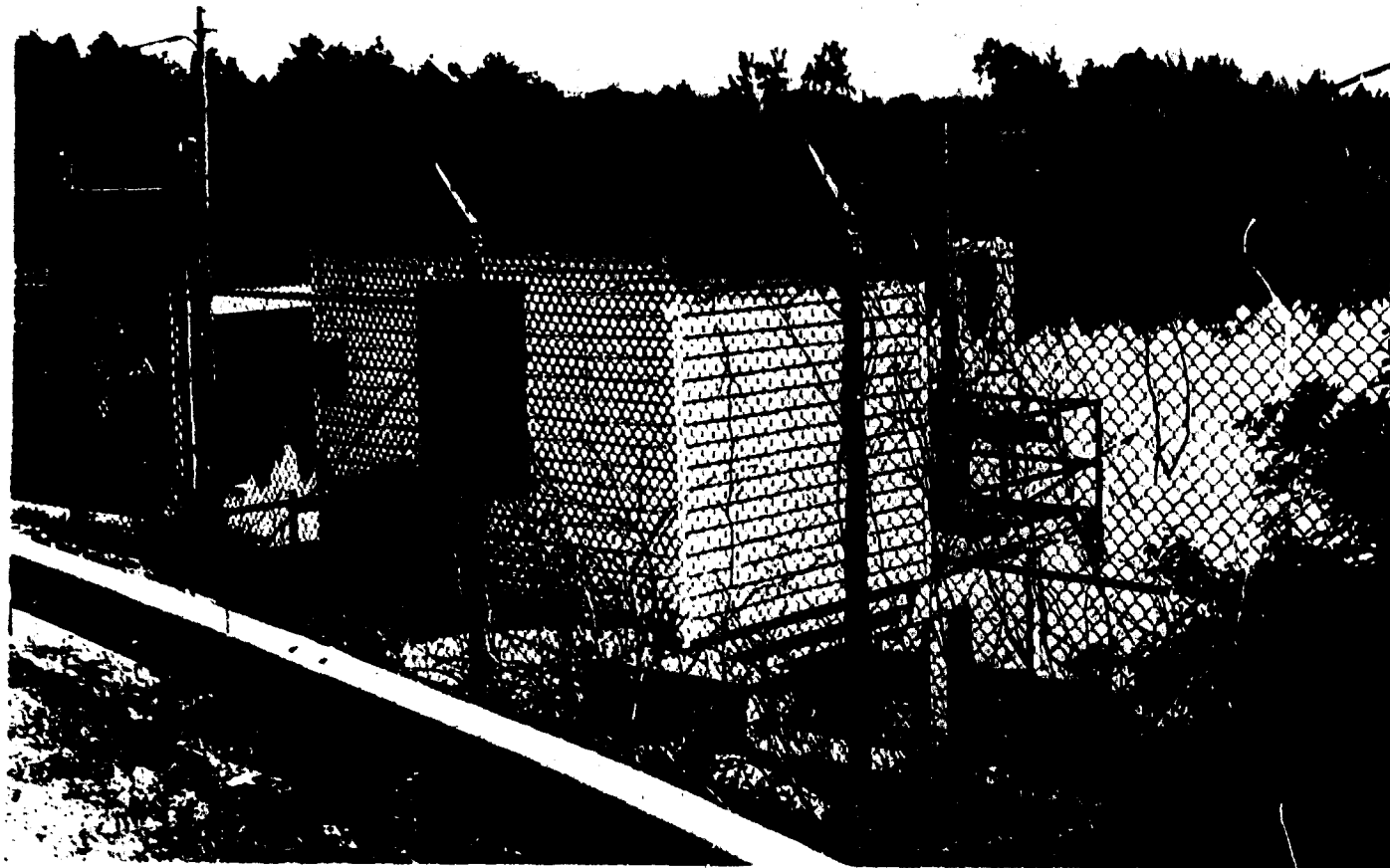
Fig. 4.3. Monitoring station at White Oak Dam.
