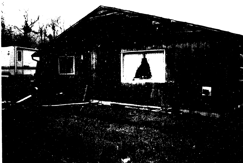
Photo 5. Exterior of home 3.
