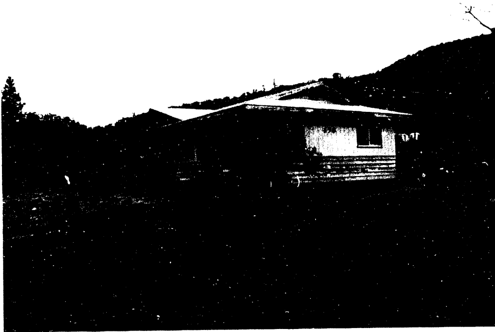
Photo 3. Exterior of home 2.
