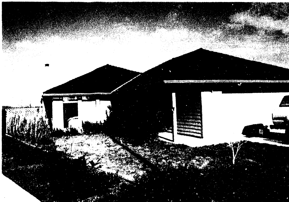
Photo 11. Exterior of home 6.
