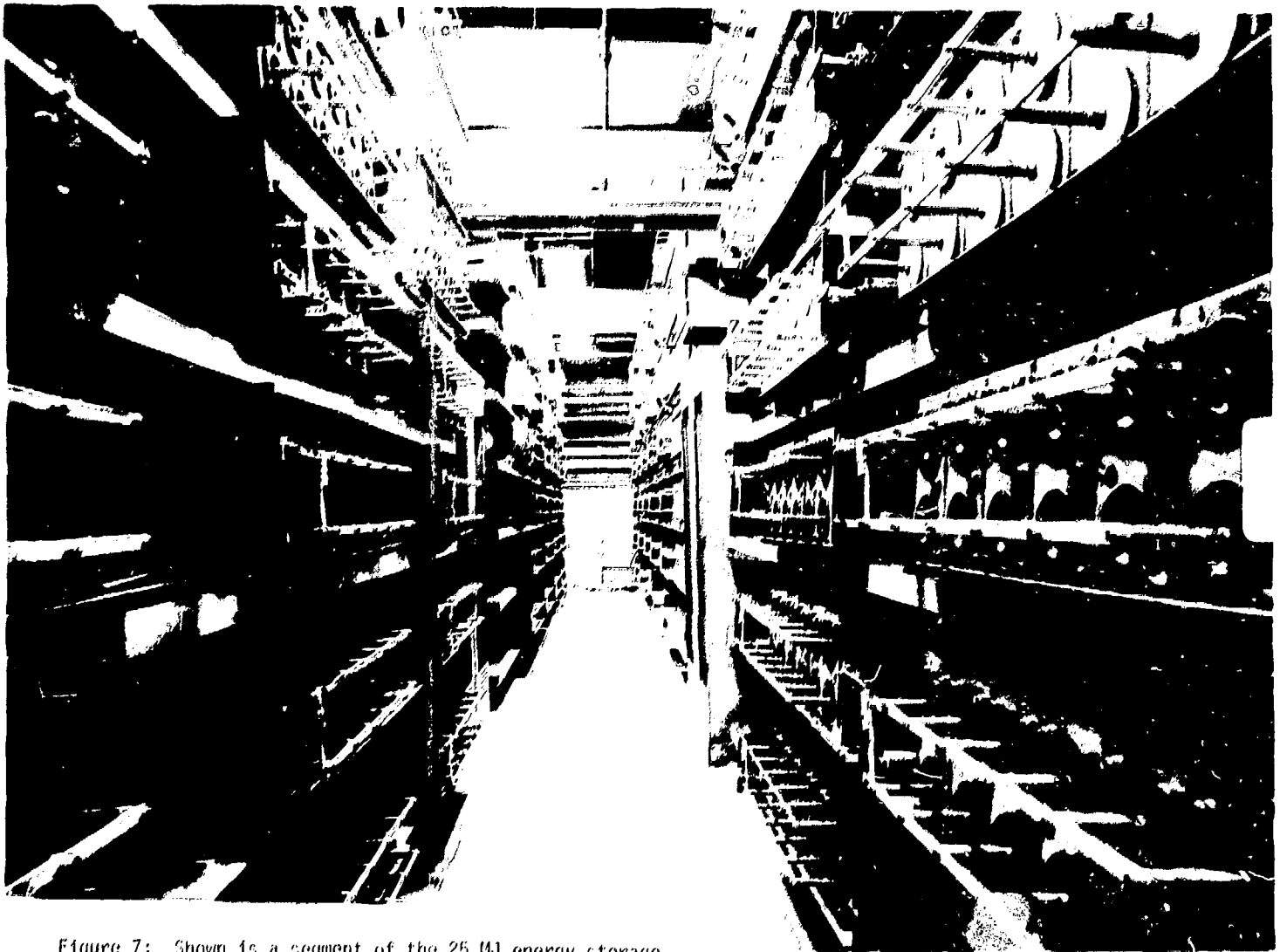
Figure 7: Shown is a segment of the 25 MJ energy storage system as installed for the Shiva laser.
