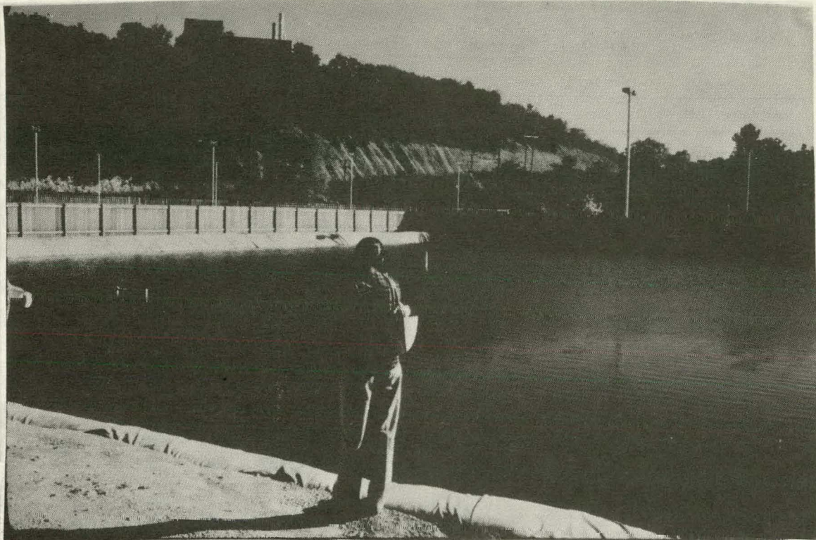
FIGURE 4. Miamisburg, Ohio - Salt Gradient Pond
