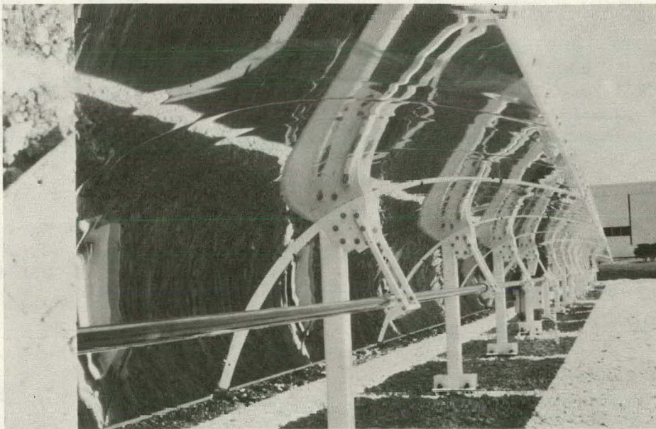
FIGURE 4. INSTALLED COLLECTOR ROW
