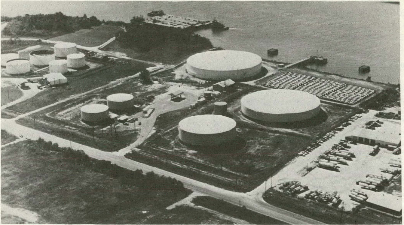
FIGURE 1. ERGON'S MOBILE BULK TERMINAL
