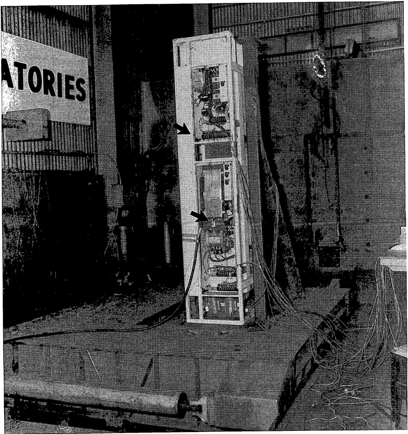
Fig. 2.3(b) X-Y axes setup for retest of MCC including seismic clips. Top and bottom arrows point to the locations of the seismic clips and the response accelerometers, respectively.
