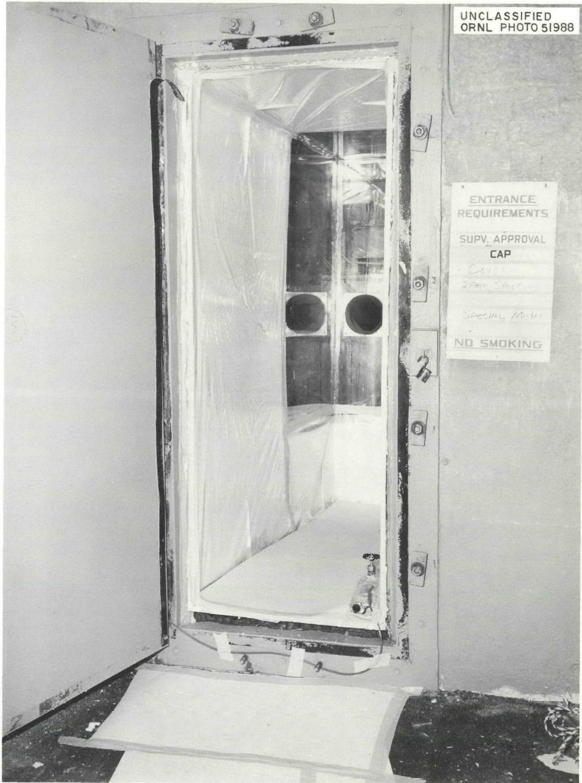
Fig. 3.1. View of greenhouse from plenum chamber.
