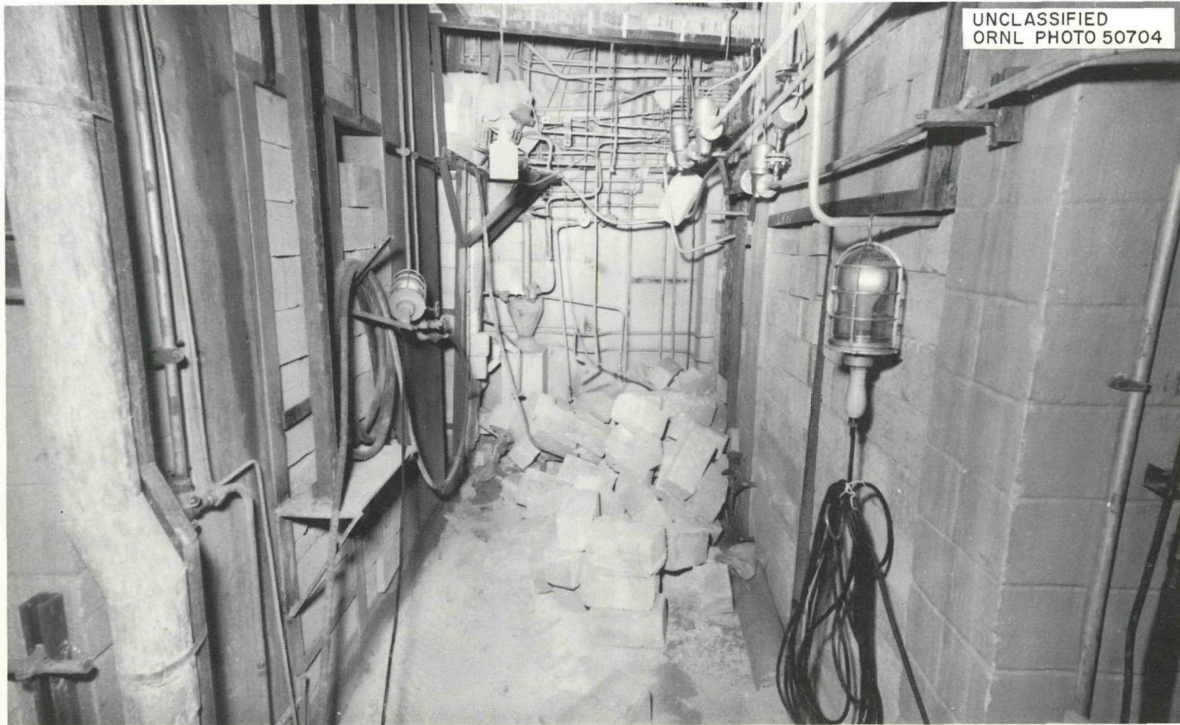
Fig. 5.1. View of cell 6 lower level prior to block and debris removal.
