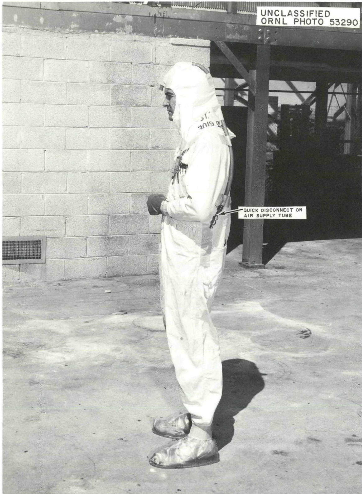
Fig. 7.2. Operator dress and air supply tube used inside plastic suit.
