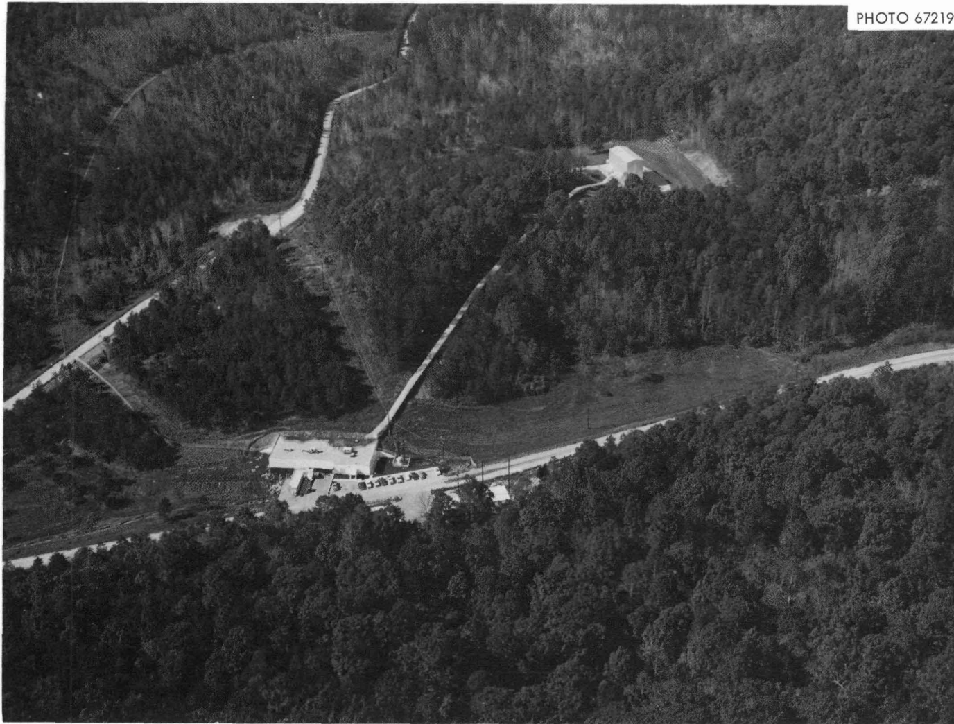
Fig. 1. Photograph of DOSAR Facility Showing Reactor Building (Upper Right) and Control Building (Lower Left).
