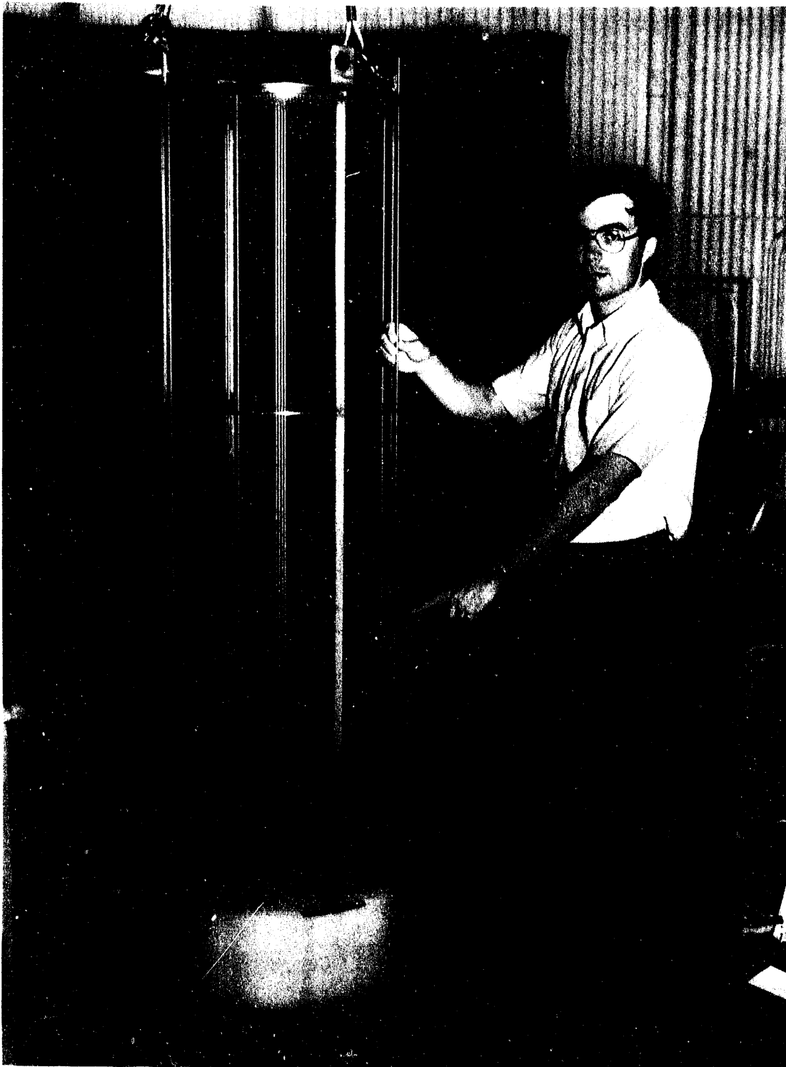
FIGURE 2.8 Photograph of Boiler Tube-Type Tank Inner Assembly
