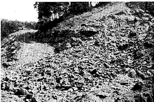
Fig. 32. Blasted rock from PB-6A.
