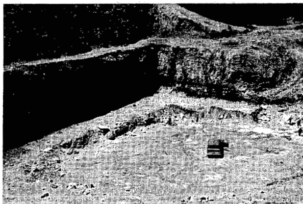
Fig. 21. PB-4 after excavation of fractured rock.
