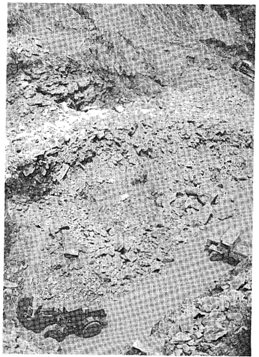
Fig. 46. PB-8 during excavation (from left rear).
