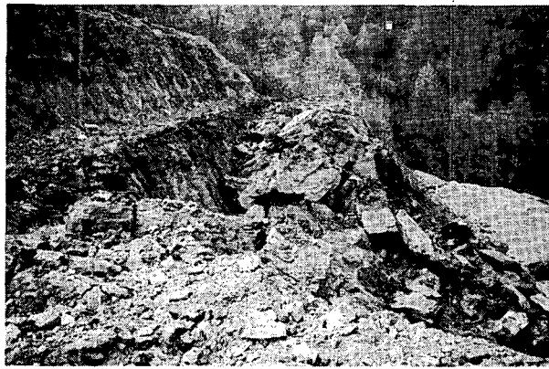
Fig. 15. PB-3 trimming/presplit, rear wall.
