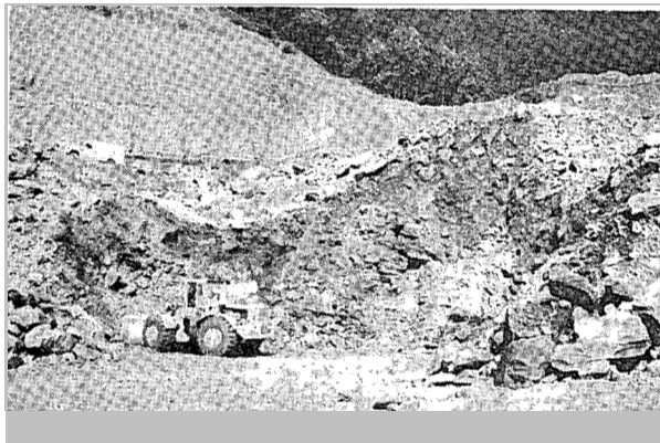
Fig. 42. PB-7 during excavation.
