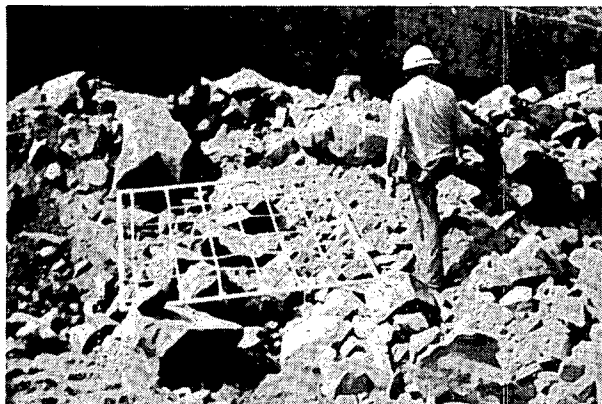
Fig. 23. Blasted rock from PB-4A (1-ft 2 grids).
