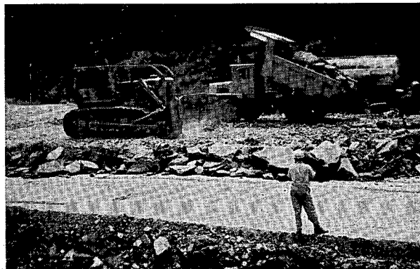
Fig. 85. Dumping and spreading test fill material.
