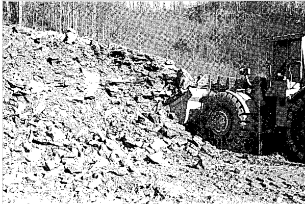
Fig. 11. Excavating from PB-1 blast.
