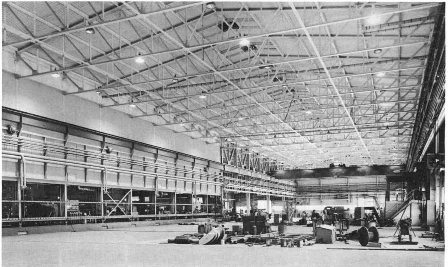
Figure 4. View of nearly completed new experimental area.
