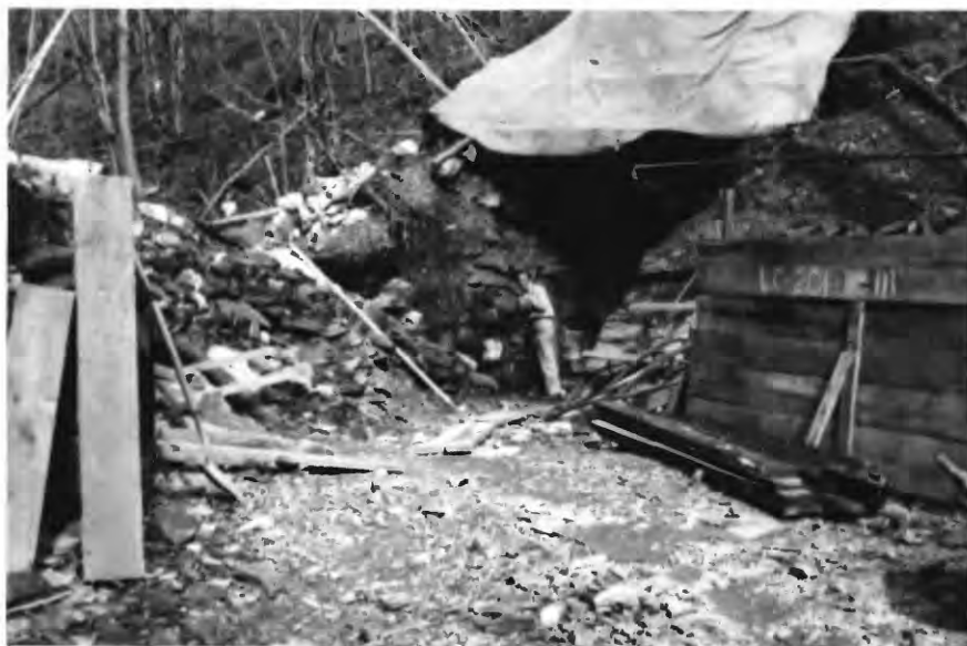
Fig. 3. View of facing cut for adit, and one of the ore bins. Photograph taken January 24, 1949.
