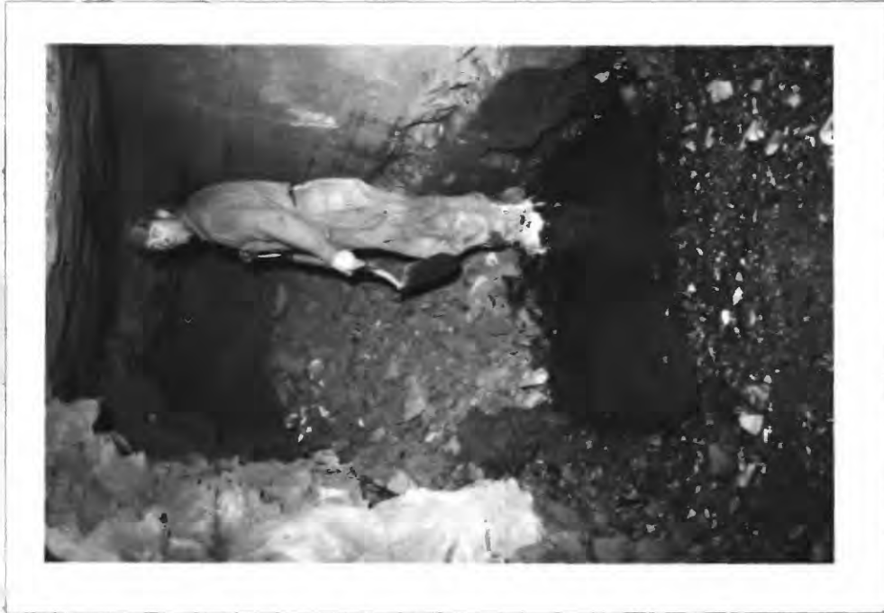
Fig. 10. Back of adit, February 8, 1949. Note joint face on right, and bed in Top Black left standing in back. The roof is the hard bed in the nodule layer.
