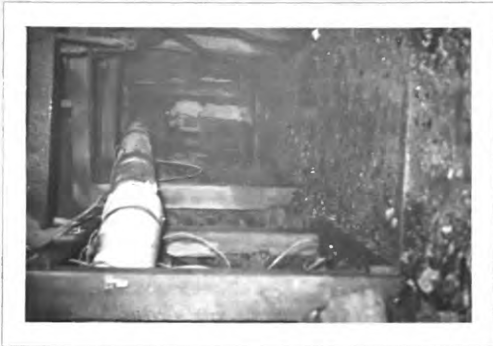
Fig. 9. View of adit from portal, showing tubing for ventilation, and timbering. January 24, 1949.
