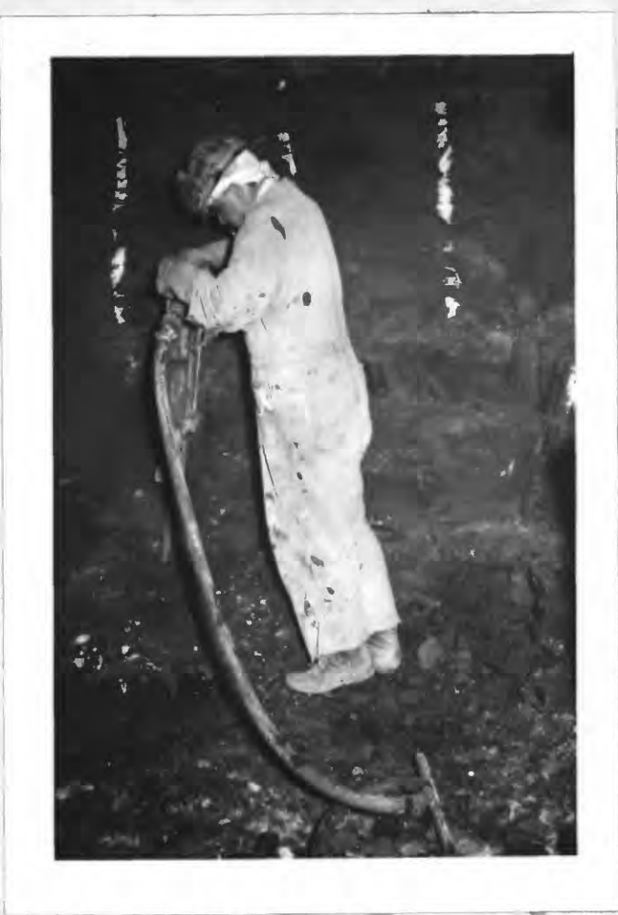
Fig. 5. Smoothing face with paving breaker, January 24, 1949.
