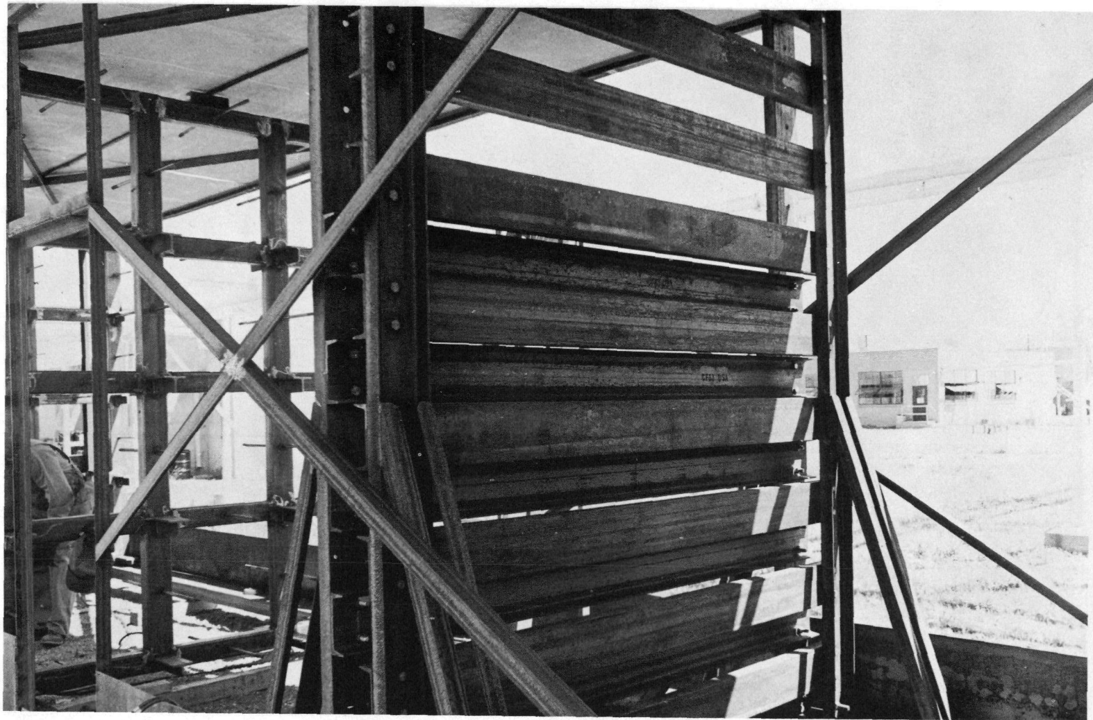
FIGURE 7 Construction of Channel Baffle
