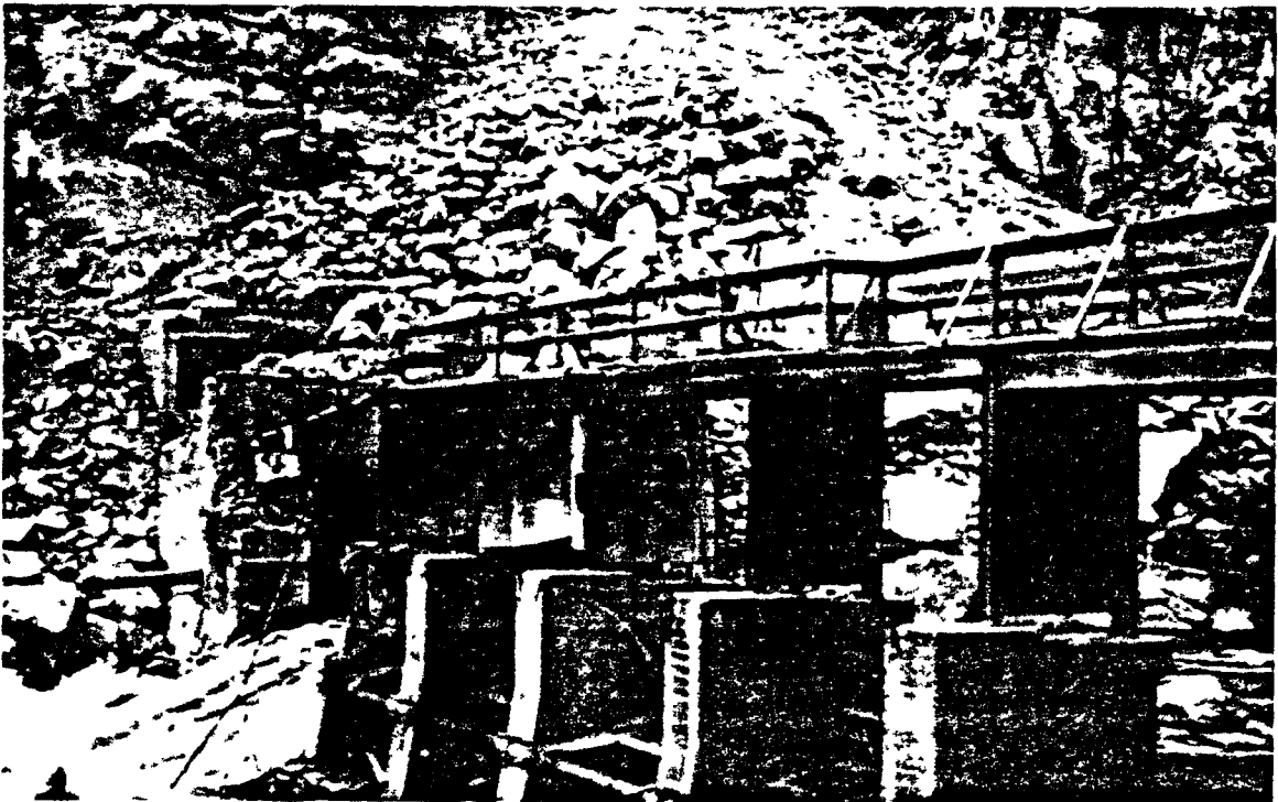
Fig. C.3—Damage to diversion dam caused by a landslide following Arvin-Tehachapi, Calif., earthquake, July 21, 1952. (Pacific Gas and Electric Company.)
