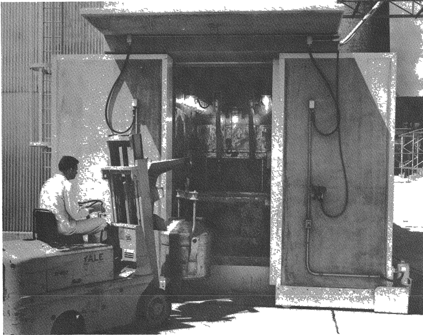
Fig. 44—Loading area of multi-kilocurie loading cell, Remote-control Cell Building, 3029, Oak Ridge.
