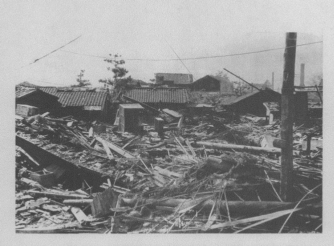
Fig. 20--(3H). Houses destroyed at Higashi-ura, Dunbara (2,000 meters). This area was partly protected from blast by Mount Hiji. The collapsed structures in the foreground represent the appearance of the city after the blast and before it was reached by the flames. The heavy tree beams were responsible for trapping many persons who were subsequently burned to death by the uncontrollable fires. (Photo File # HB 451.)
