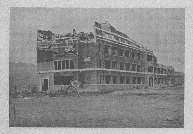
Fig. 17b--(3N). Chinzei Middle School after the explosion. This building was 500 meters from the center. (Photo File #NB 113c.)
