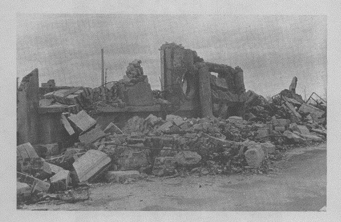
Fig. 25--(3H). Brick building with load-bearing walls. Shima Hospital. This structure was within 50 meters of the point above which the bomb exploded. Note the huge lethal fragments in which the building has collapsed. There were no survivors. (Photo File # HB 424.)
