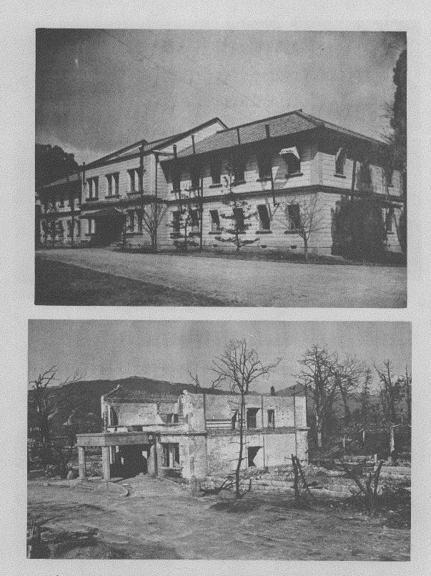
Fig. 16 a, b--(3H). Hqs. Chogoku Army (800 meters) before and after bombing. (A portico has been added since the first photograph). The wooden wings have collapsed and burned. The brick central section has partly collapsed. (Photo File # HB 113 a, b.)
