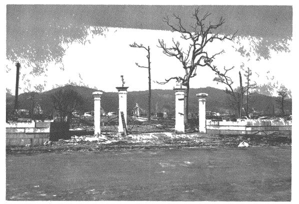
Fig. 17 a, b--(3H). Prefectural Office (900 meters) before and after bombing. The wooden structure has collapsed and burned. Note displacement of the heavy granite blocks of the wall. (Photo File # HB 112 a,b.)
