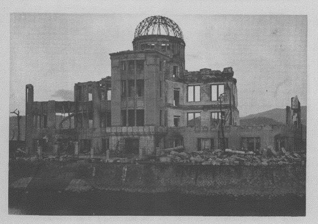
Fig. 15 a, b--(3H). Commercial Museum (300 meters) before and after bombing. Collapse of massive brick and reinforced concrete walls. (Photo File # HB 118 a, b.)
