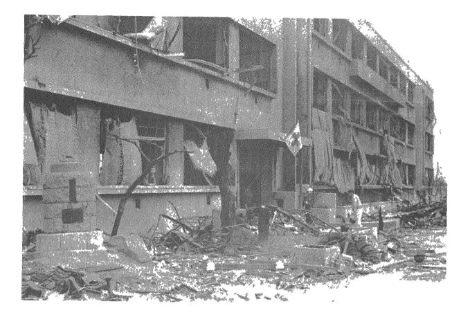
Fig. 47--(3H). Fukuromachi School (700 meters). This building, not far from the center of the explosion, was one of the few left standing in the area. It was put to immediate use as an aid station. Note mats used for shelter. (Photo File # HH 207.)
