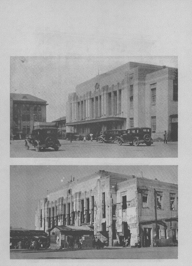
Fig. 12 a, b--(3H). Hiroshima Railroad Station (1800 meters) before and after bombing. Structure stands, but roof has collapsed (see figure 12 c). (Photo File # HB 105 a, b.)
