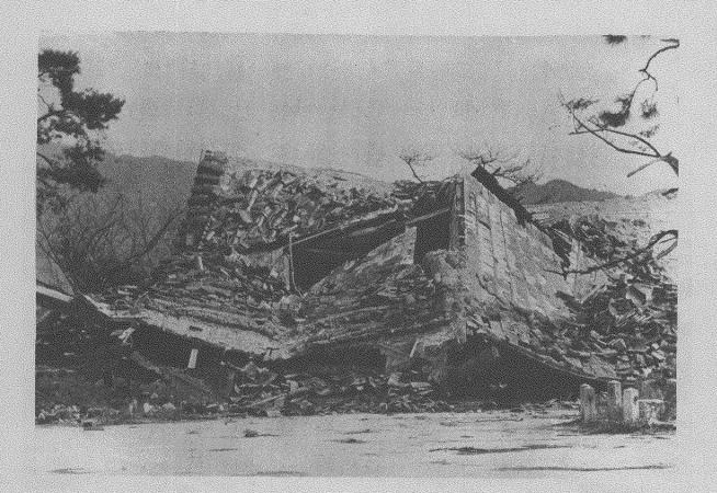
Fig. 21--(3H). A typical Japanese building at Hijiyama (1800 meters). The great longitudinal tree beam that supported the roof can be seen. The heavy pantiles are also visible. (Photo File # HG 411.)
