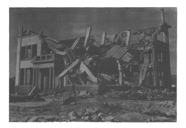
Fig. 23--(3H). The Hiroshima Gas Company Building (200 meters). Collapse of brick-faced, reinforced concrete wall. Columns still stand. (Photo File # HB 421.)
