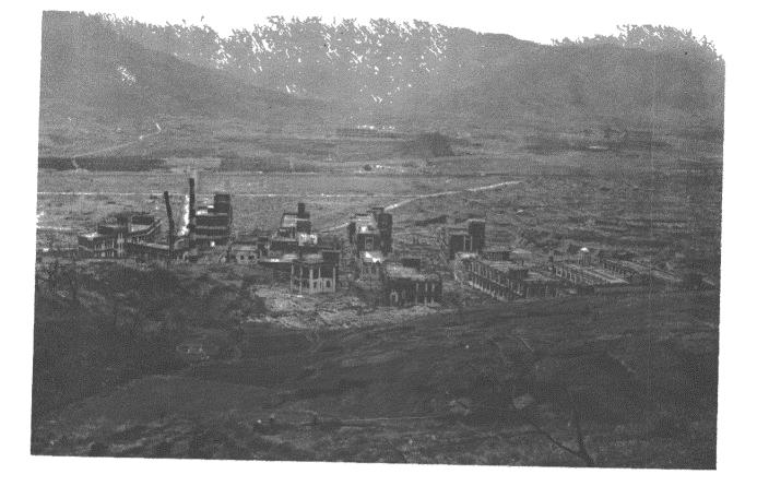
Fig. 18b--(3N). The Hospital of the Nagasaki Medical College after the bombing. Only the reinforced concrete buildings remain. (Photo File #NB 105b.)
