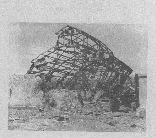
Fig. 19--(3H). "Mass distortion" of a steel-framed factory shed (600 meters). The entire building leans away from the center of the explosion. The metal sides have been crushed against the frame like paper blowing in the wind. (Photo File # HB 415.)
