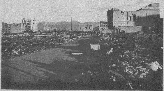
Fig. 10 a, b--(3H). Komiya Street (750 meters) before and after bombing. The archlike heavy lamp posts have fallen. One lies at the left of the lower photograph. (Photo File # HB 117 a, b.)
