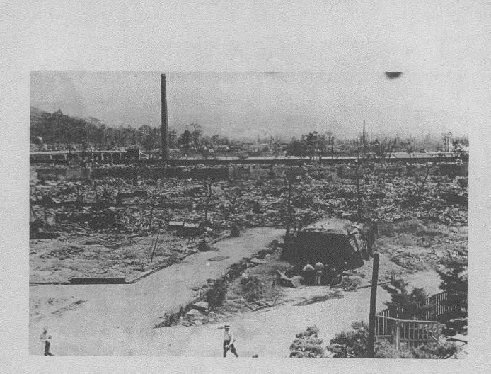
Fig. 26--(3H). An air raid shelter of excavated, timber-supported, board-roofed, and dirt-covered construction remains intact amid the surrounding devastation (1100 meters). These shelters were almost deserted at the moment of explosion. After the bombing they served as temporary housing. (Photo File # HH 157.)
