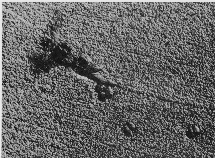
Figure 8 T10163 25X Indentations in Crack C. Enlargements of Area Shown in Fig. 7.
