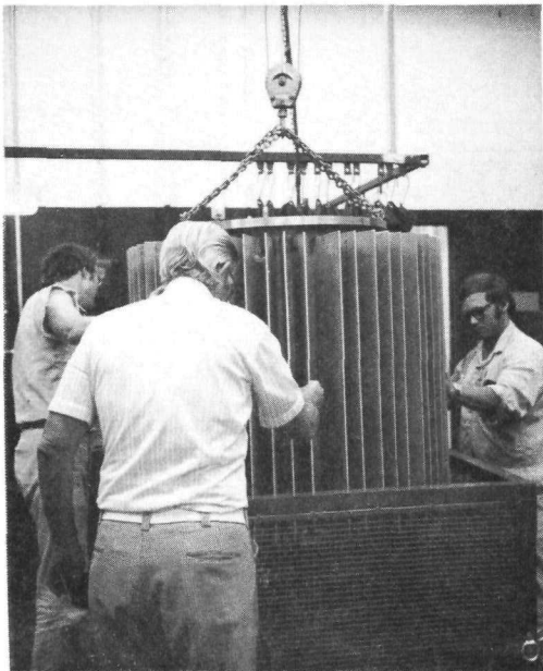
FIGURE i-16 - The finned cask is being installed in the carrier.
