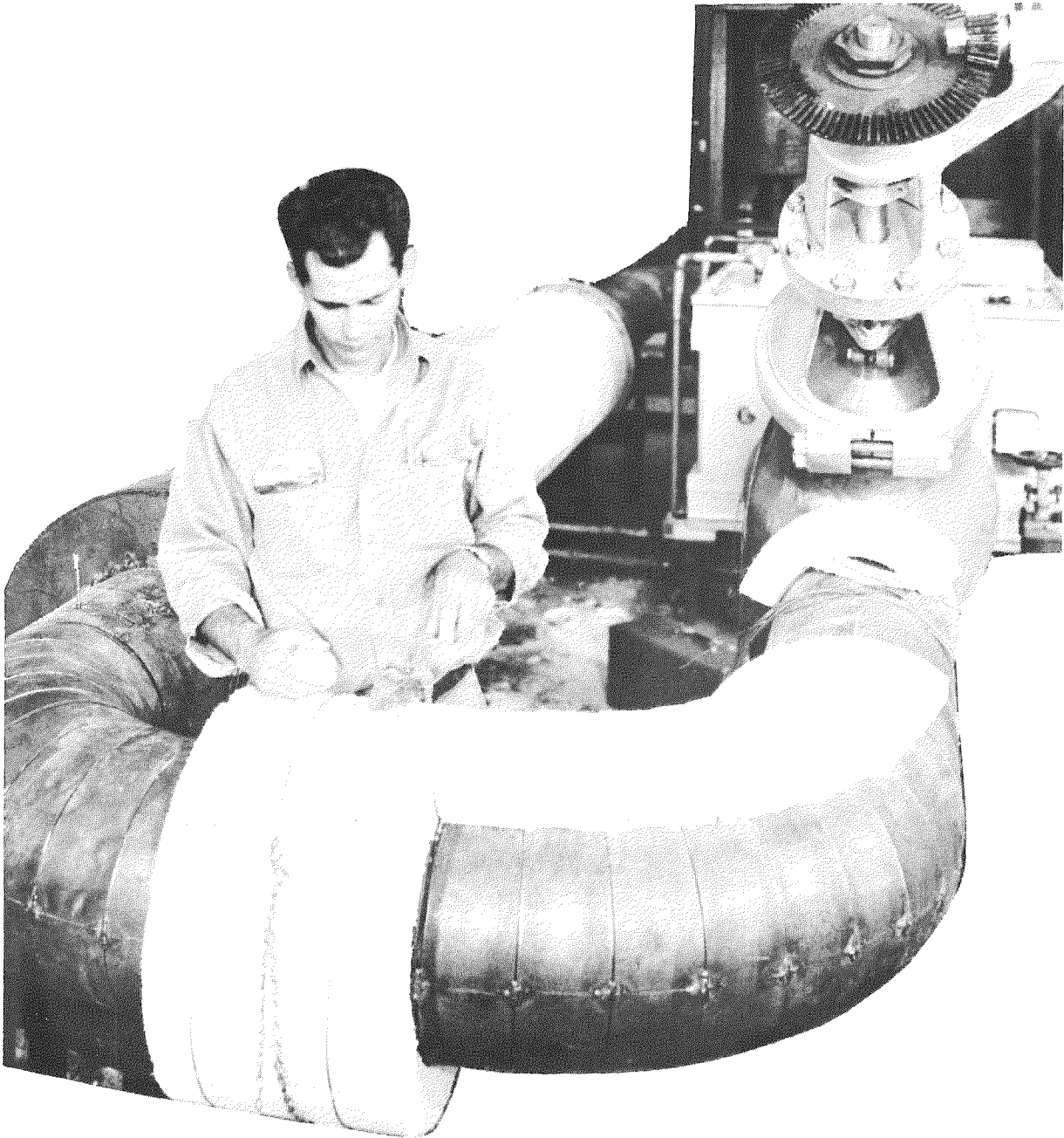
FIG. 14 THERMAL INSULATION BEING APPLIED OVER TACK WELDED CARBON STEEL CLADDING
